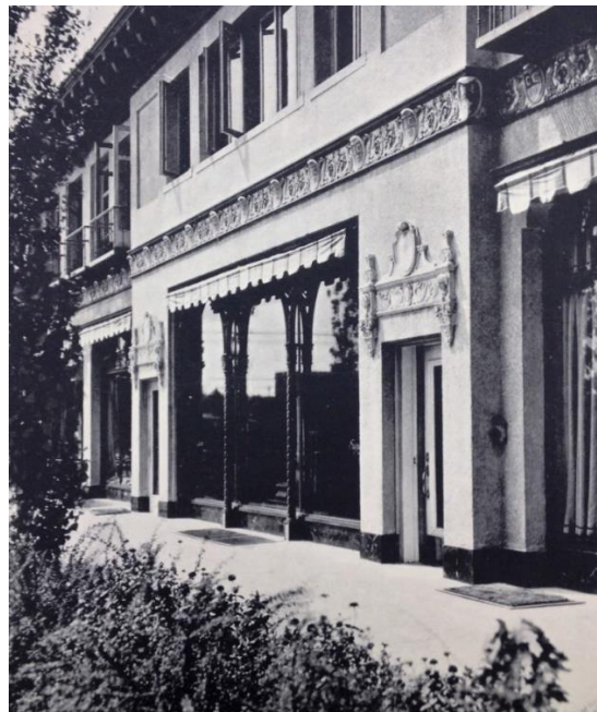
Figure 23: The exterior of the Mill Creek Building. J. C. Nichols Company Scrapbooks, SHSMO-KC
