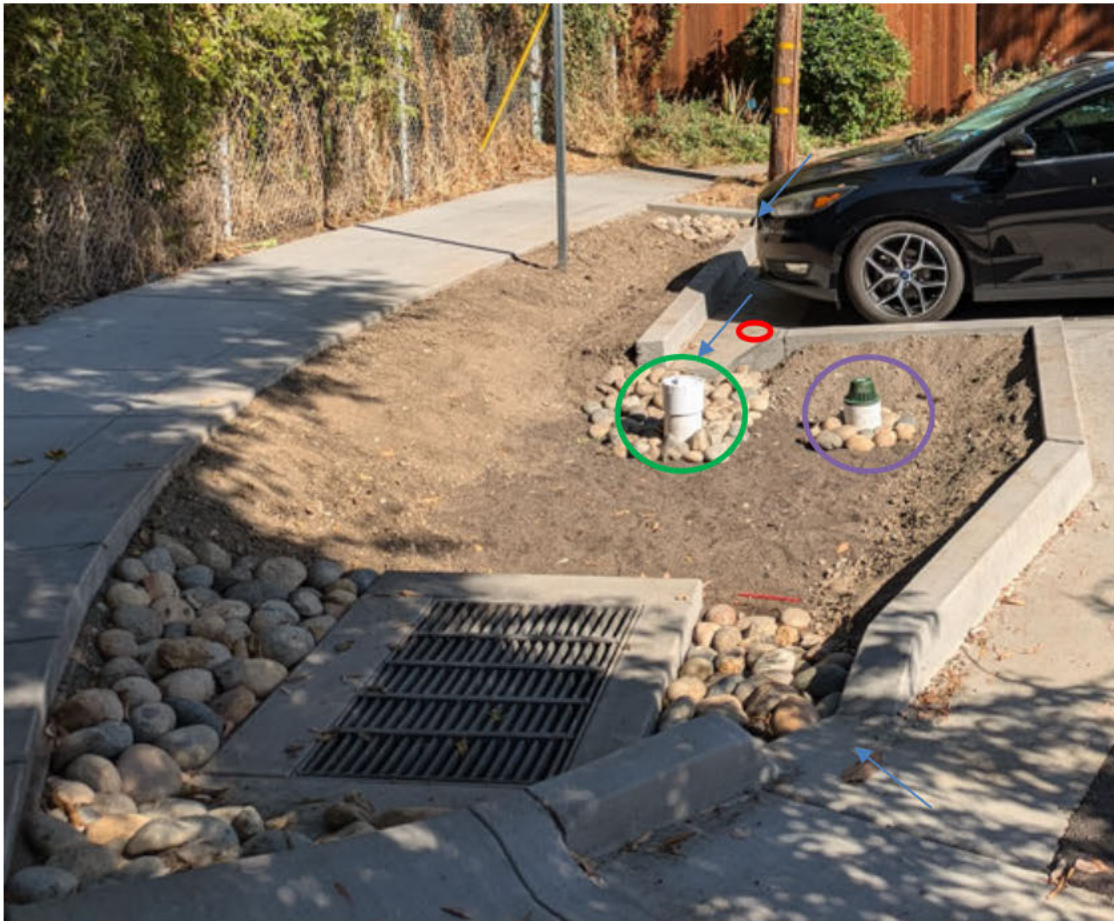
Figure 24: Photo of the bioretention facility before planting with labels showing the influent (red circle) and effluent (green circle) observation wells and the air drainage/clean out portal (purple circle).
