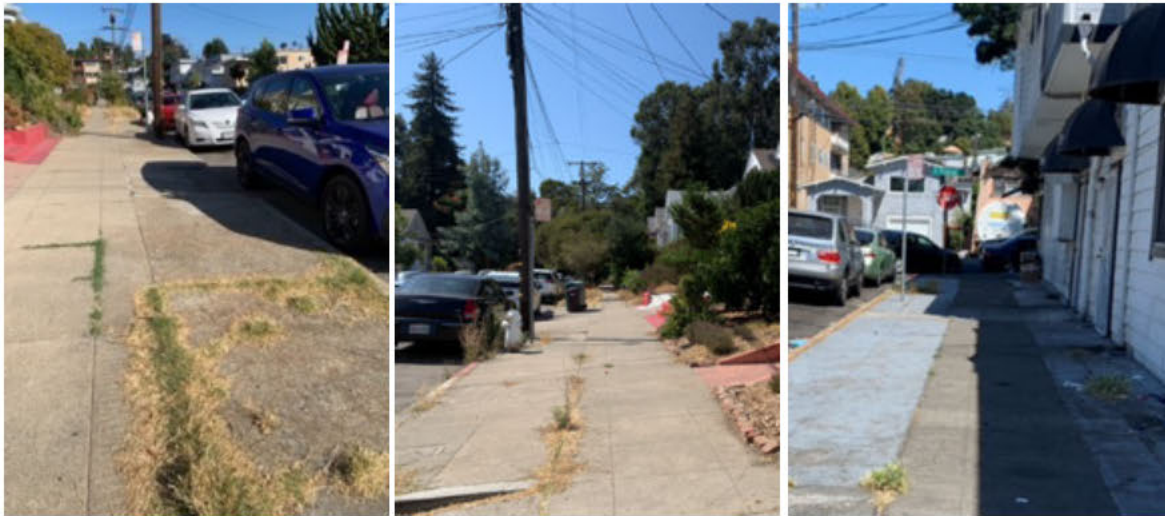
Figure 16: Previous concrete-filled planting strips along the block. Credit: Therese Peffer
