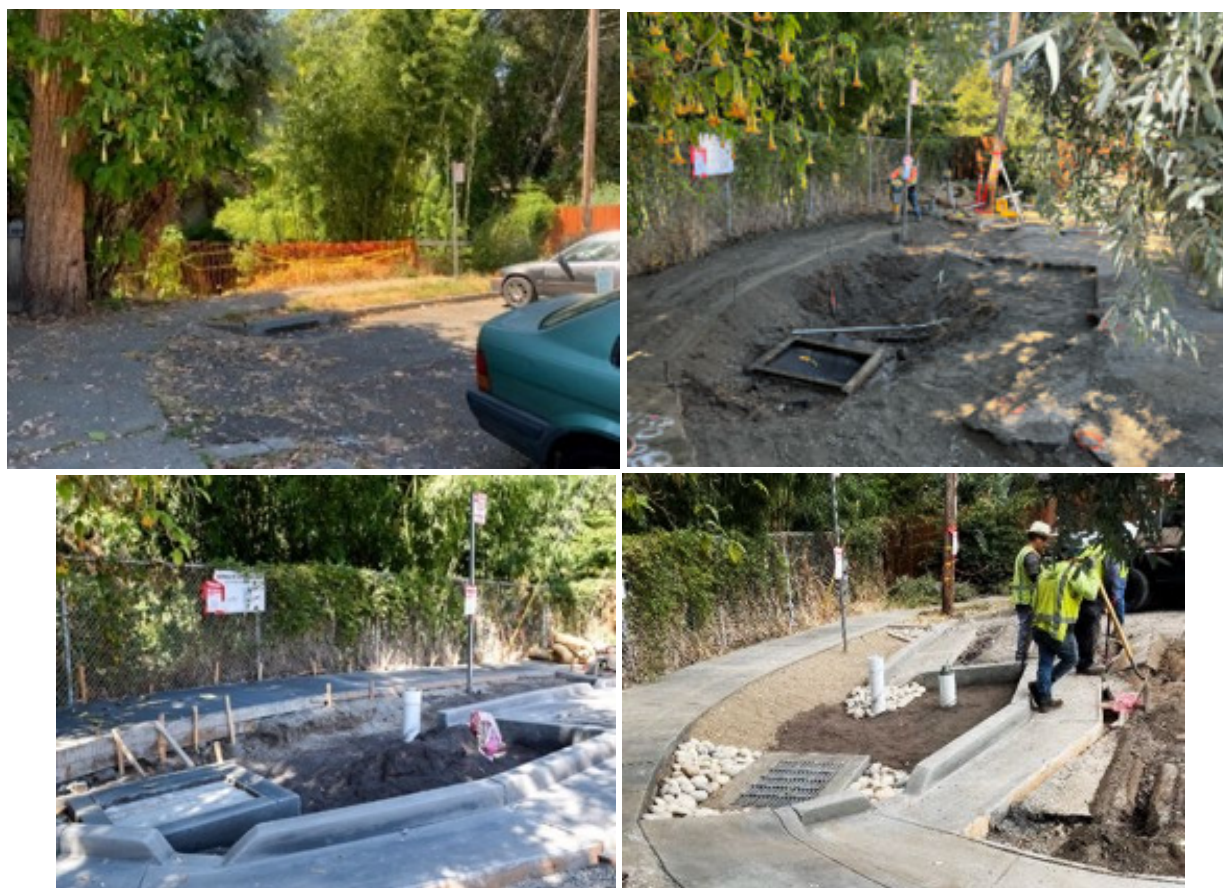
Figure 8: Construction timelapse of the stormwater bioretention facility. Credit: Therese Pfeffer, Haixin Guo, and Keith O'Hara
