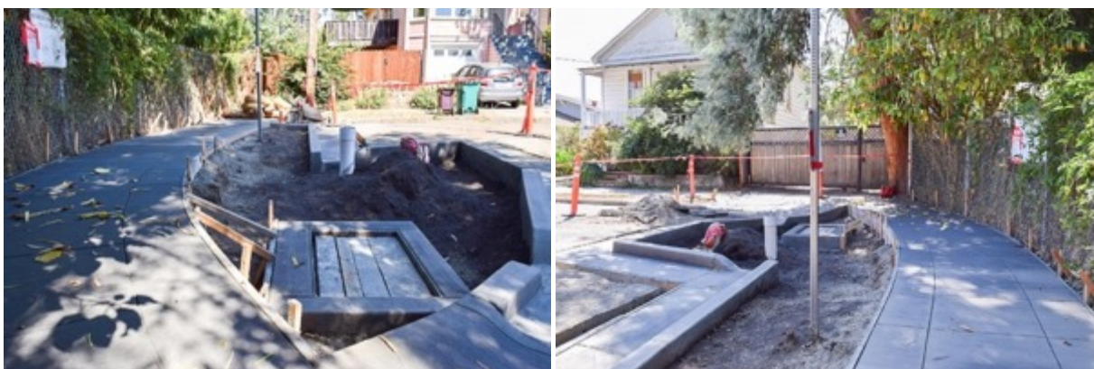
Figure 9: The west and east ends of the stormwater facility under construction. Credit: Haixin Guo
