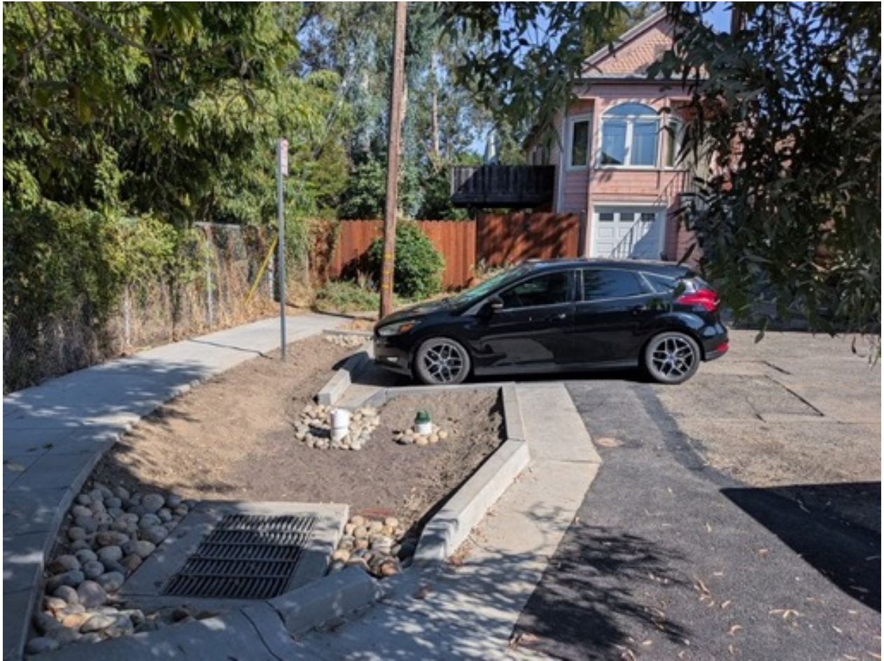
Figure 11: The nearly completed stormwater bioretention facility, with the exception of the painted red curb and planting. Credit: Phillippe Phanivong
