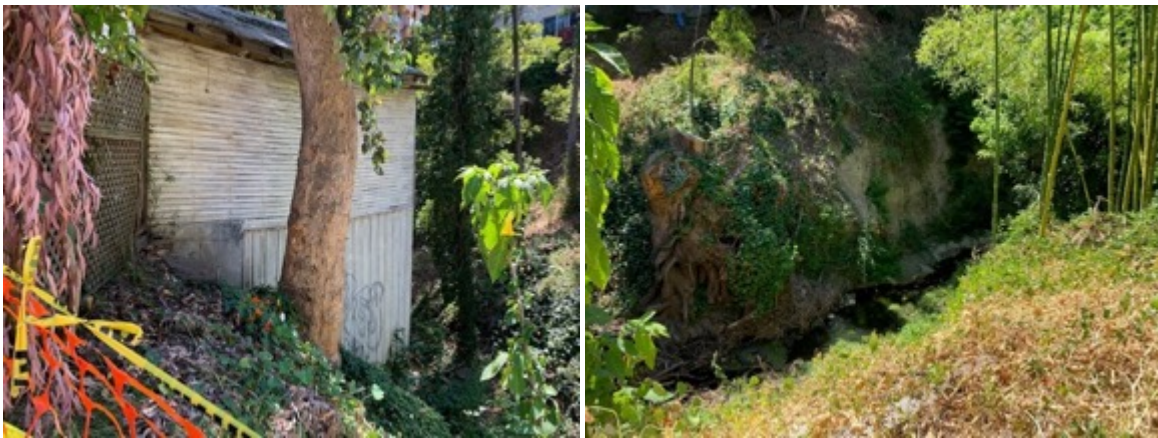
Figure 4: The end of the block overlooking Sausal Creek, (top) showing the pre-construction condition (single curbside drain) and (bottom) showing the steep slope down to the creek, emphasizing the erosion concerns exasperated by stormwater runoff. Credit: Therese Peffer
