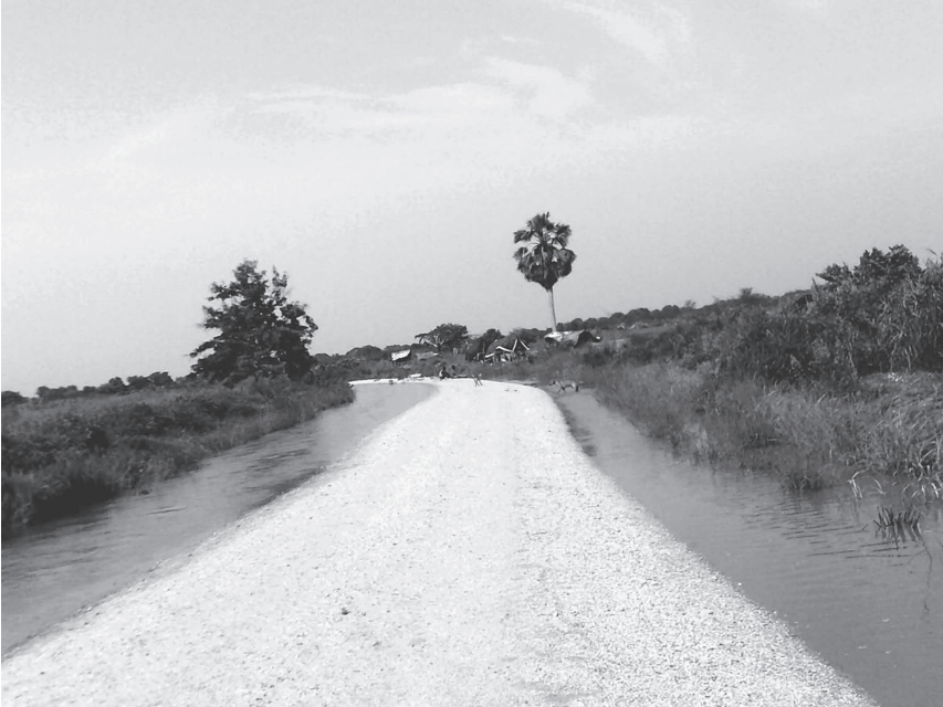
FIGURE 6.2. The road from Makaani to Gama during masika (the long rainy season). The mvumo (African fan palm) stands at the location of Fatuma’s and Thabiti’s farm. Photo by Hasani, February 2016.
