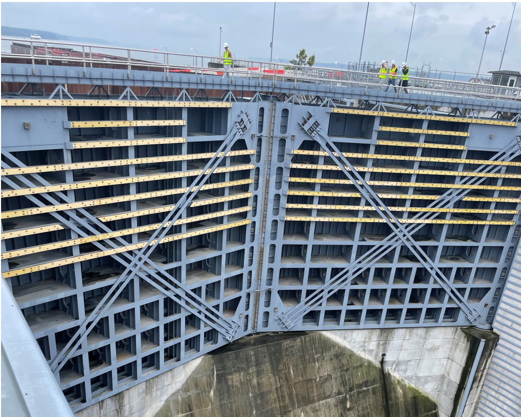
Figure 2.11. A miter gate in the dewatered state.
