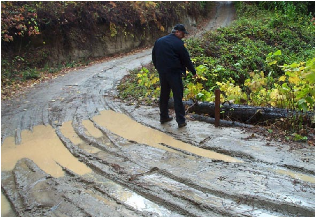
Figure 2. Use of unsurfaced roads in the winter can lead to erosion and sediment delivery to streams. Photo: Courtesy Angela Wilson.
