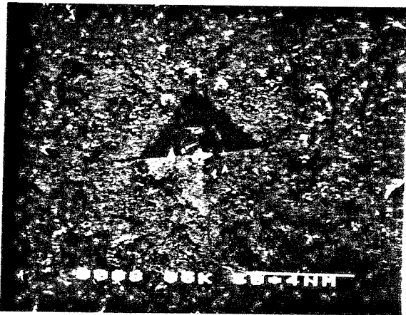
Fig 4.10 Development of a System of cracks (1-year old specimen)
