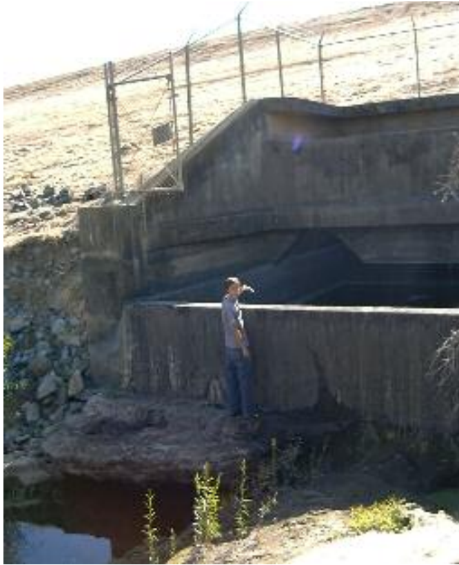
Figure Four: Downstream Face of Marsh Creek Reservoir dam
