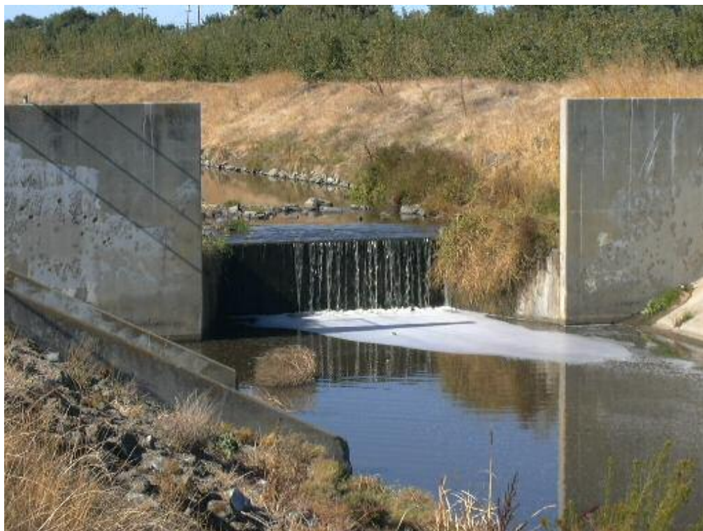
Figure Three: Drop Structure on Marsh Creek, looking Upstream
