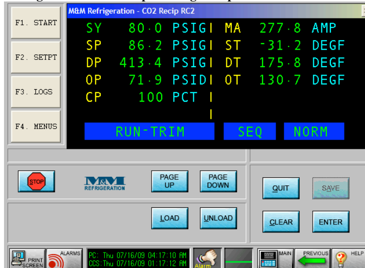
Figure 20: RC2 Reciprocating Compressor Status Screen
