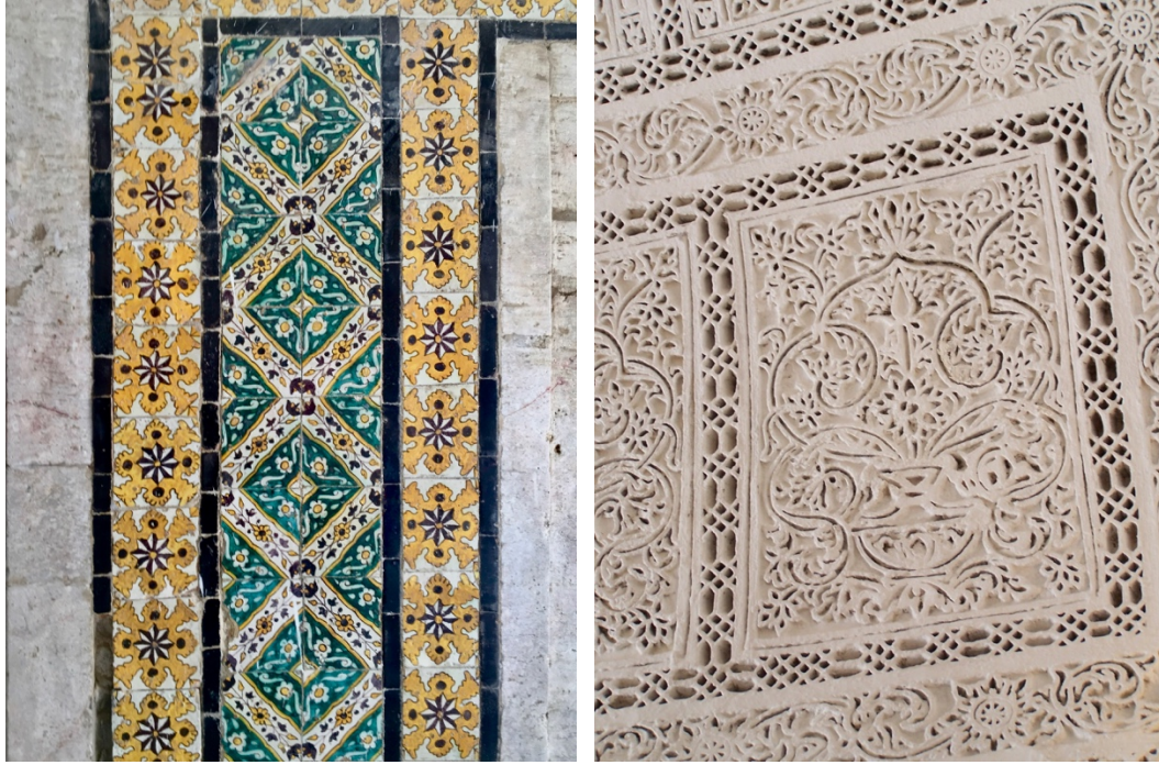
Figure 45 (left) zelāj ceramic tiling, (right) an example of naqsha haddīd , stucco work “carved with iron”
