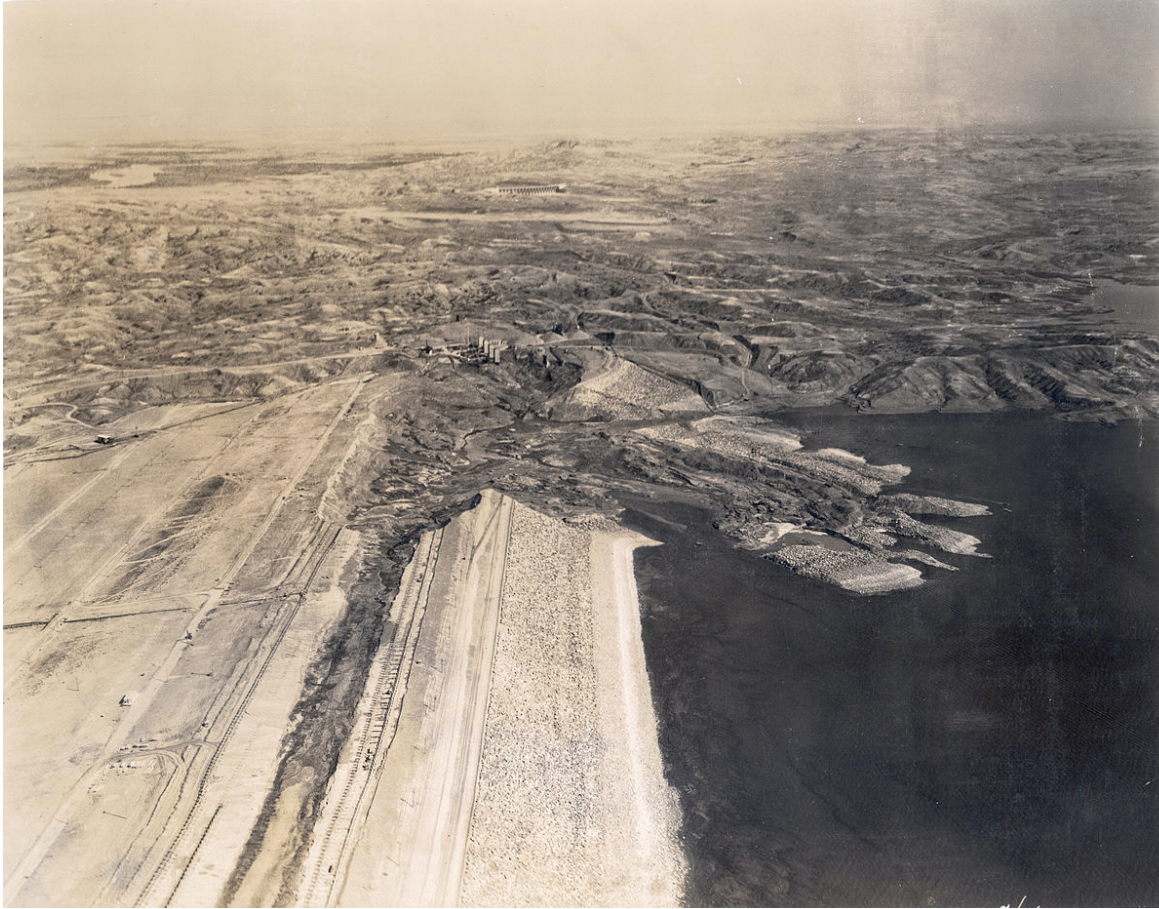
Above: Montana's 1938 Ft Peck Dam (partial) failure. The dam itself (lower left) is 250' tall at its crest with a 500-acre area. Inevitably, where control of water was concerned, manipulation of land was the medium for its realization, sometimes grandiosely. Army Corps of Engineers.
