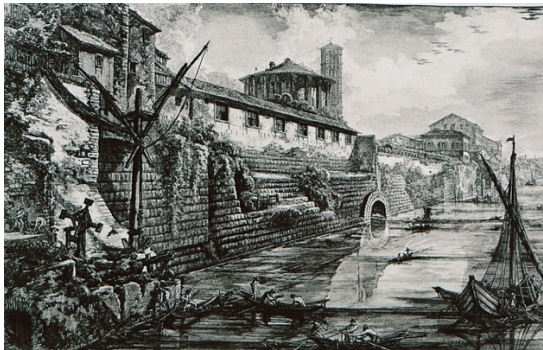
Form and Void: The 6 th Century BC Cloaca Maxima of Rome's outfall at the Tiber River (Left) is still in existence and partially functional, thus sometimes referred to as the least expensive infrastructure ever built. While essentially invisible, its construction nonetheless involved extensive earthwork. (R): 3 rd Century BC Adenaen Serpent Mound in Midwestern America: a notable earthwork of altogether different form and intent. University of San Francisco.
