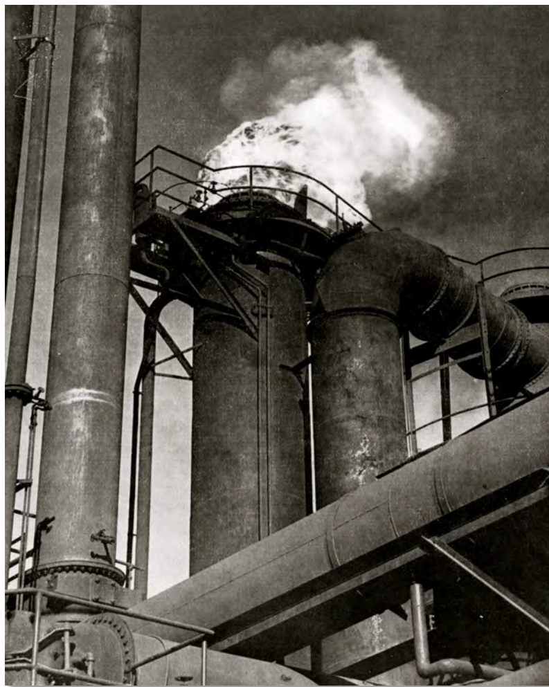
Figure 3 – First commercial scale methane reforming unit, Pittsburg, CA, ca. 1932. 54
