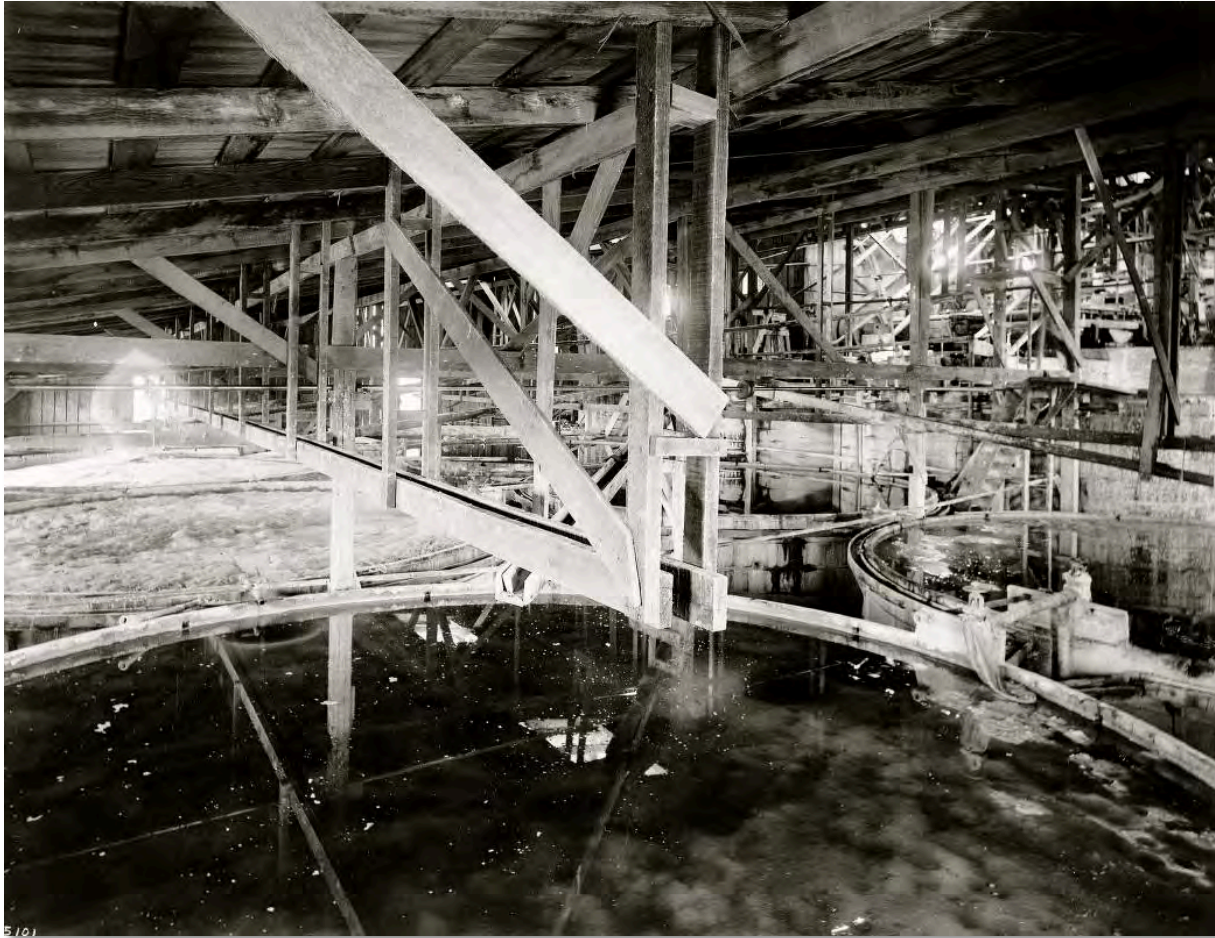
Figure 9 - Cyanide tanks, Karma Mining Company, Mojave mining district, Kern County, ca. 1900. Courtesy of the USC Digital Archive 131
