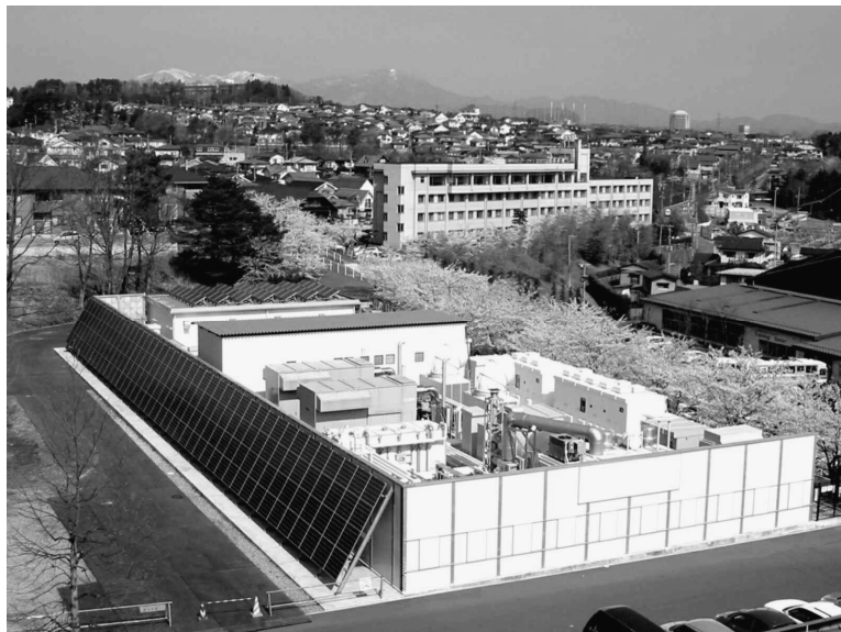
Figure 6: Sendai microgrid installation. (source: NTT Facilities)
