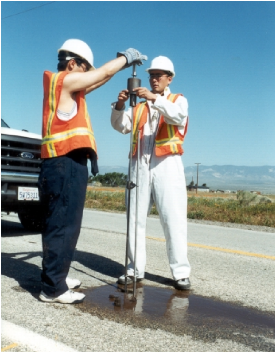
Figure 4. Crew performing DCP measurements on State Route 138.
