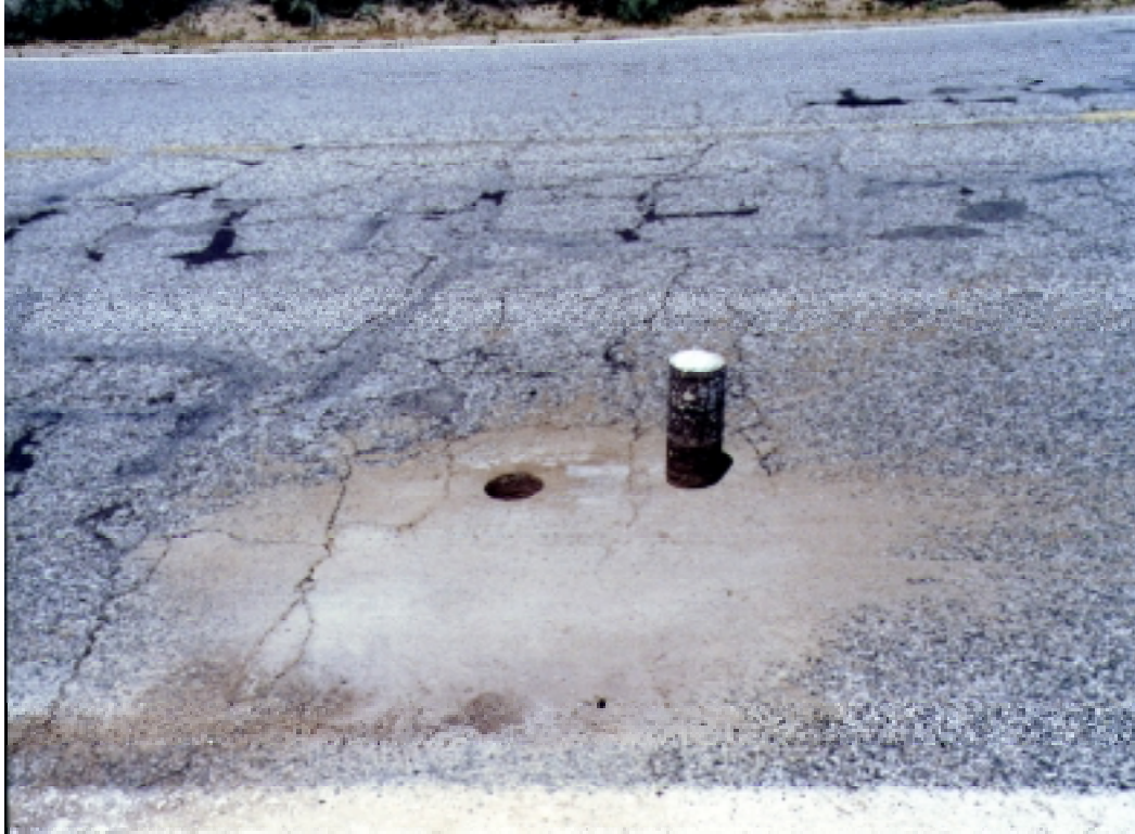
Figure 2. Typical pavement core for State Route 138.
