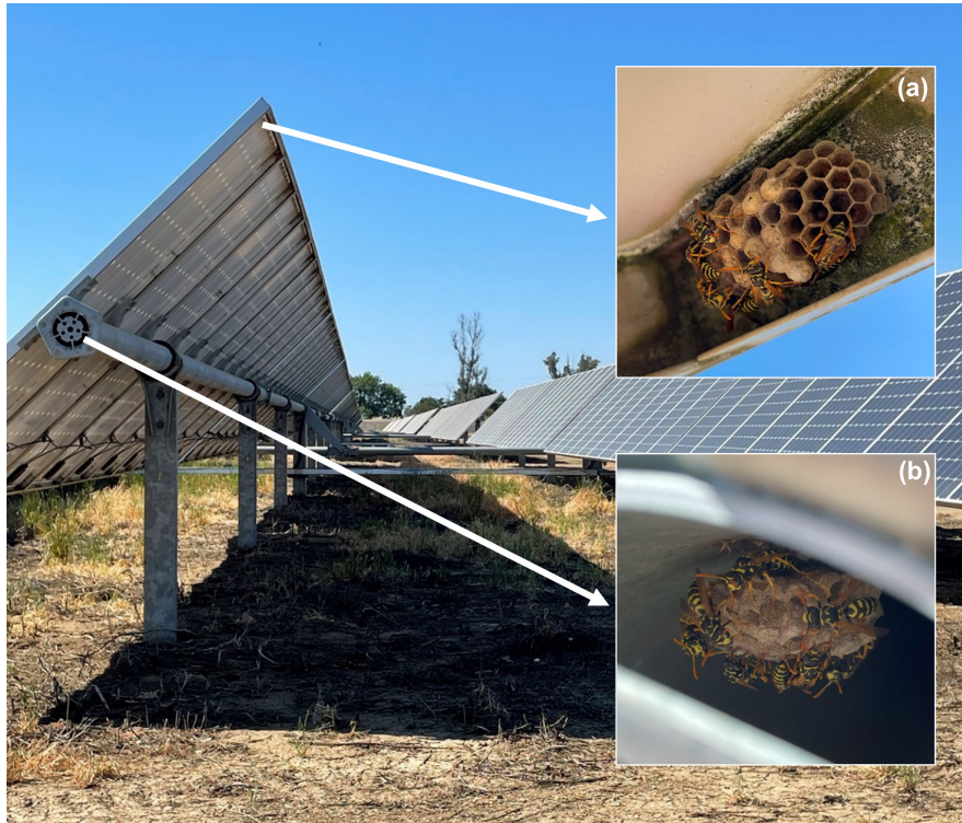
FIGURE 2 | European paper wasps ( Polistes dominula ) nesting on solar infrastructure at the UC Davis solar facility (Davis, California, USA). Nests are constructed in two locations: (a) on the underside of photovoltaic panels and (b) inside metal torque tubes. Photo credit: Nicholas Tew.
