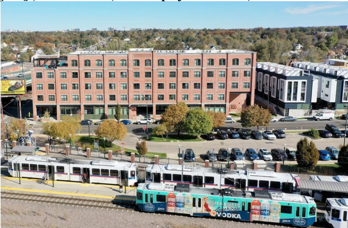
Figure 3.7: Evans Station, an eTOD project in Denver, Colorado
