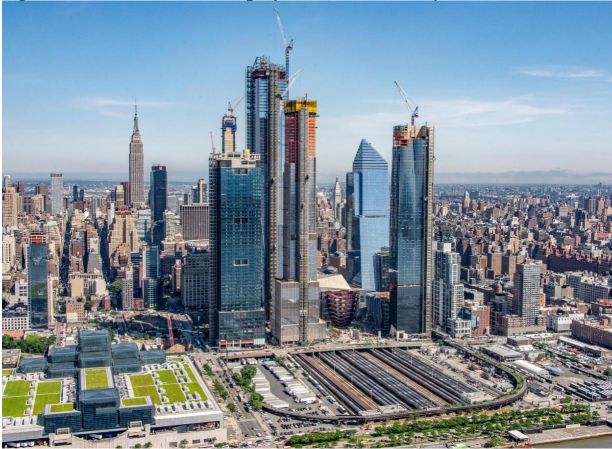
Figure 3.5: The Hudson Yards project in New York City in 2018
