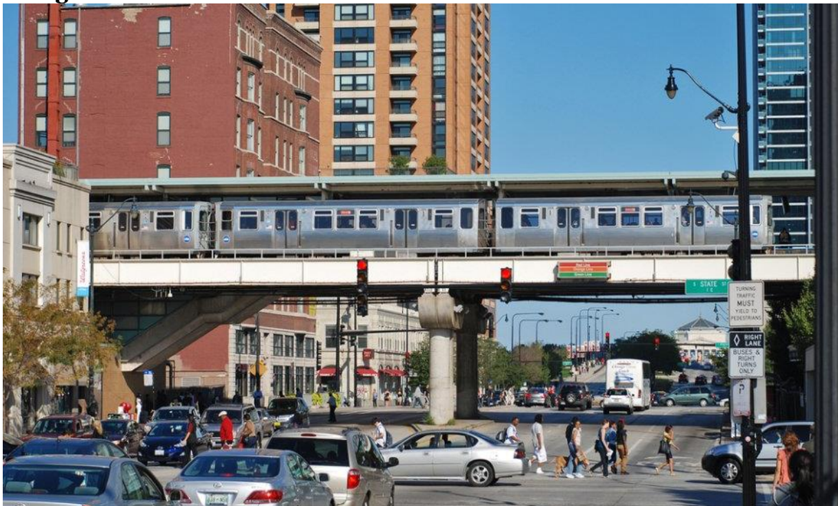
Figure 3.6: Elevated "L" Train stops at State Street and Roosevelt Street, Chicago
