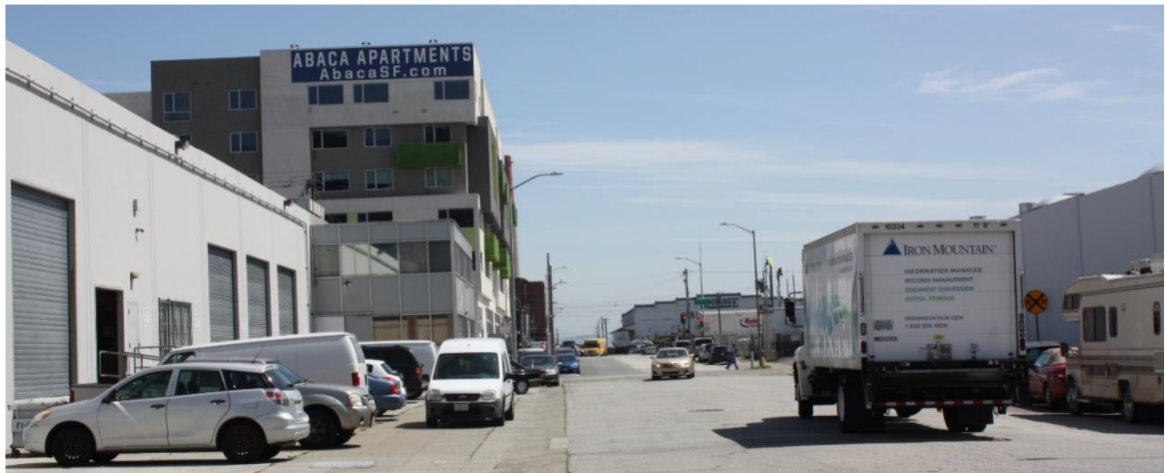
Figure 5: New residential building in industrial area
