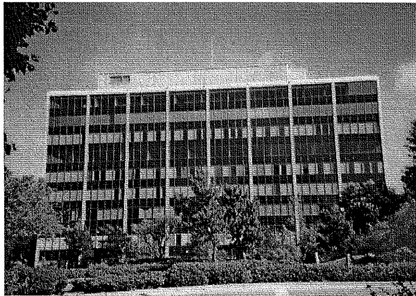
View of structure, looking in the reference south direction
