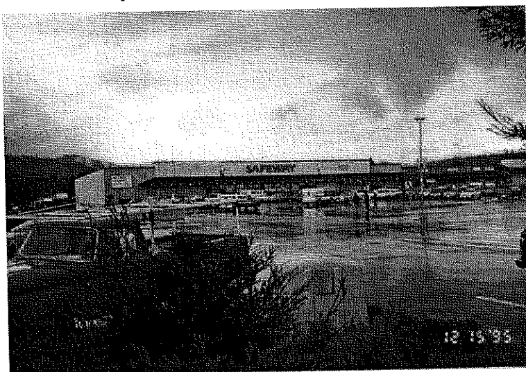
View of structure with FF in foreground
