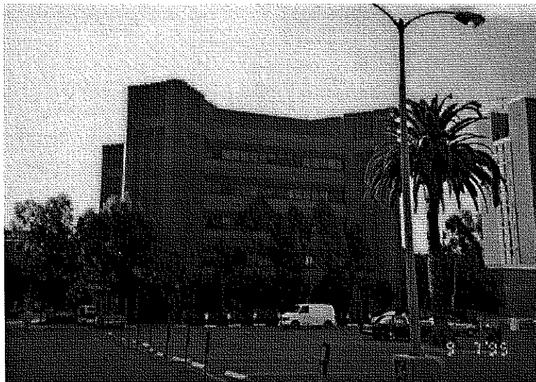
View of structure, looking south-east
