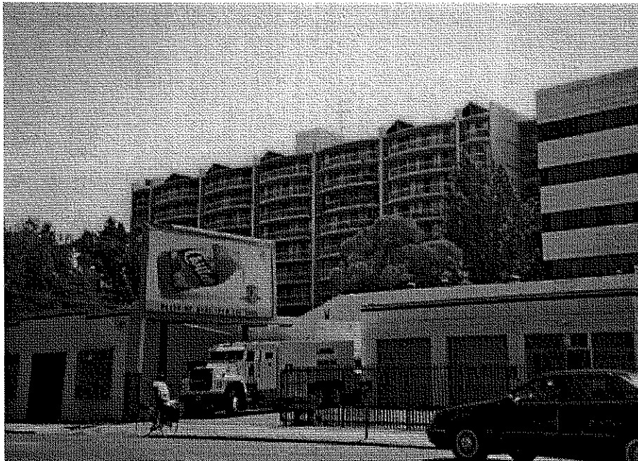
View of structure, looking south
