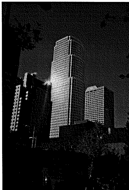
View of structure, looking north
