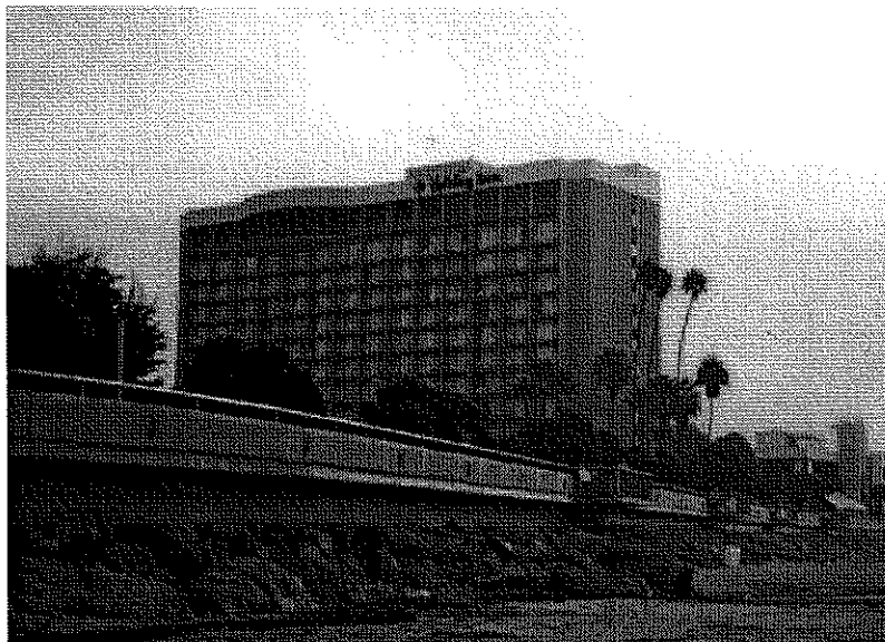
View of structure, looking north-east
