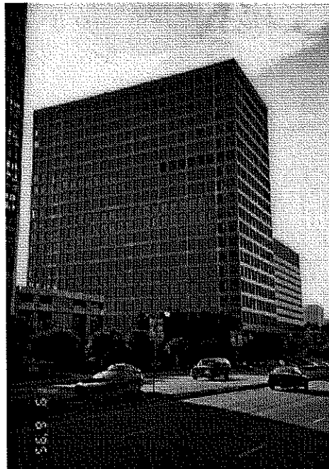
View of structure, looking west
