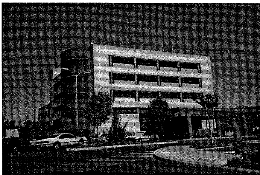
View of structure, looking north-east
