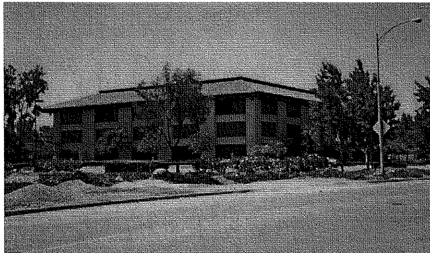
View of structure, looking south-west
