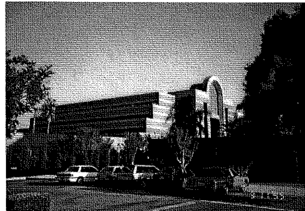
View of structure, looking south-east
