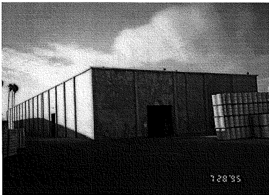
View of structure, looking north
