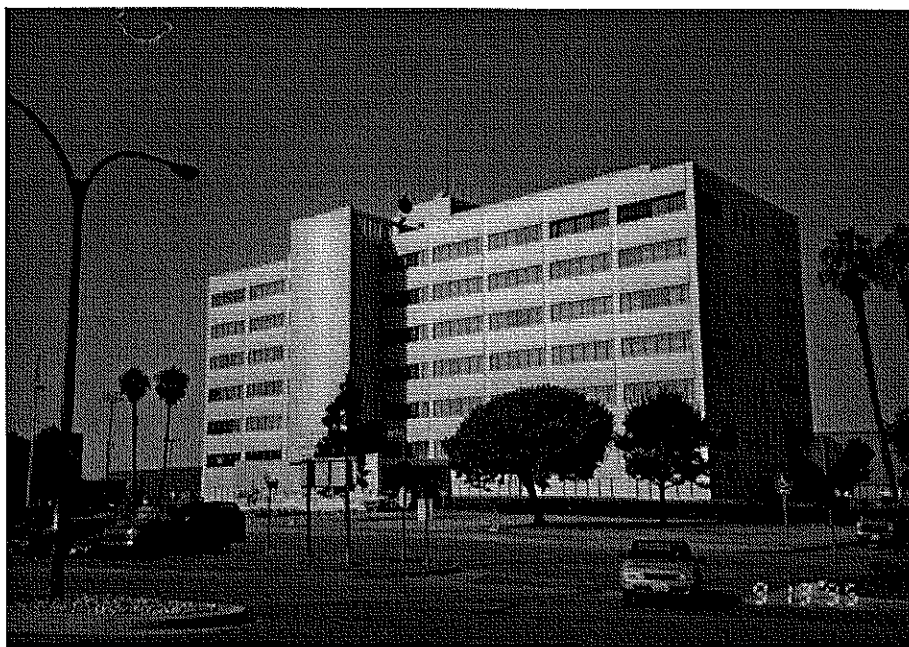
View of structure, looking south-west
