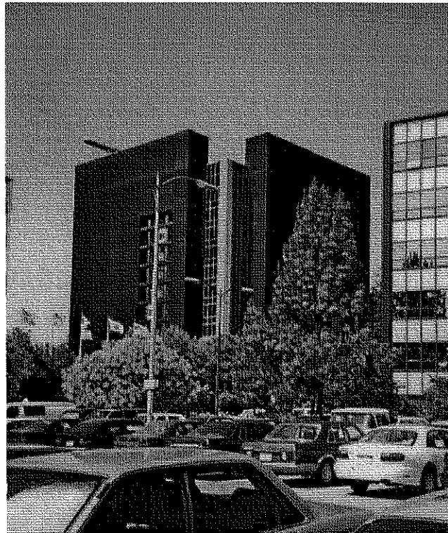
View of structure, looking north-east
