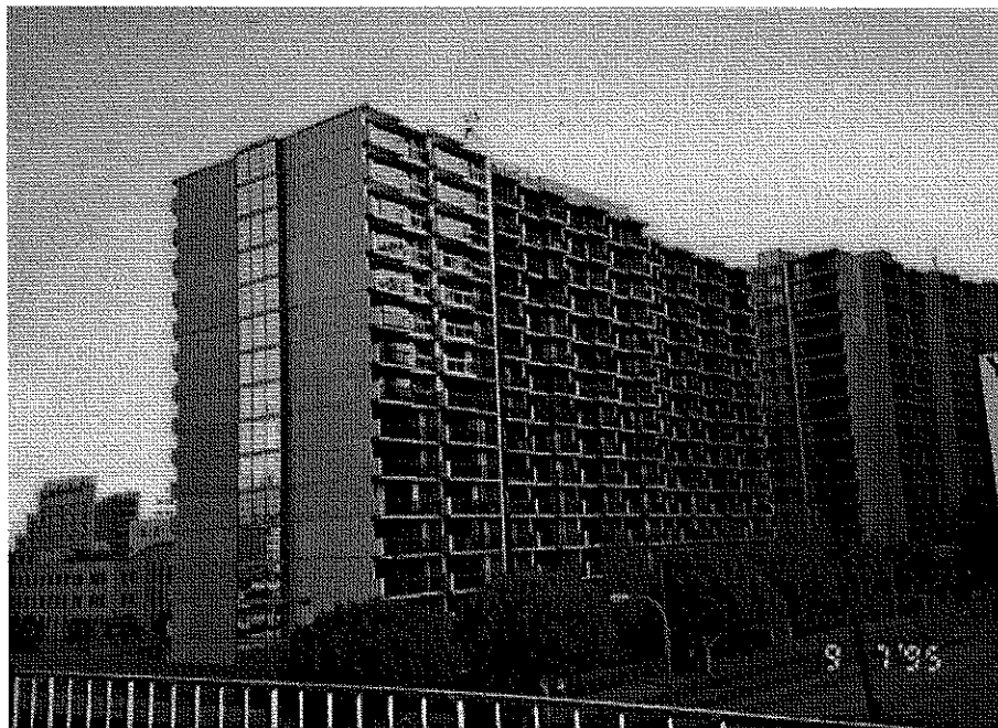
View of structure, looking north
