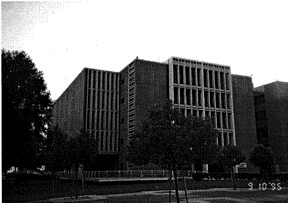
View of structure, looking south-west
