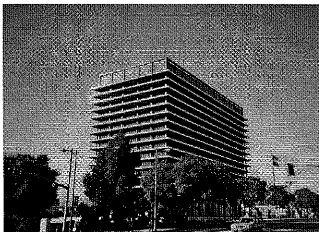
View of structure, looking north
