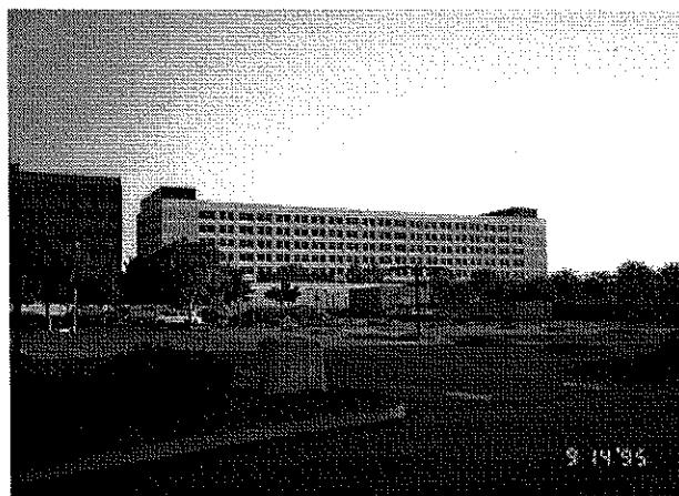
View of structure with FF2 in foreground
