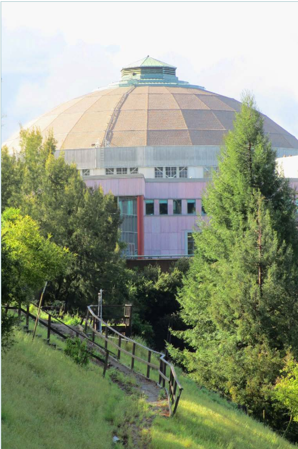
Scientists from around the world use the Advanced Light Source in Building 6.
