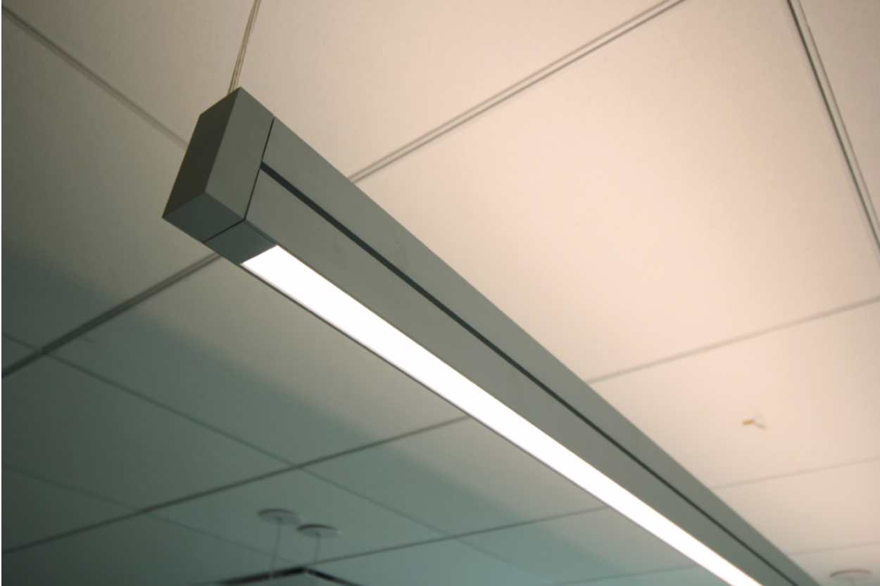
Figure 3.1 - Photo of the pendant LED light fixture installed in FLEXLAB manufactured by Vode Lighting.
