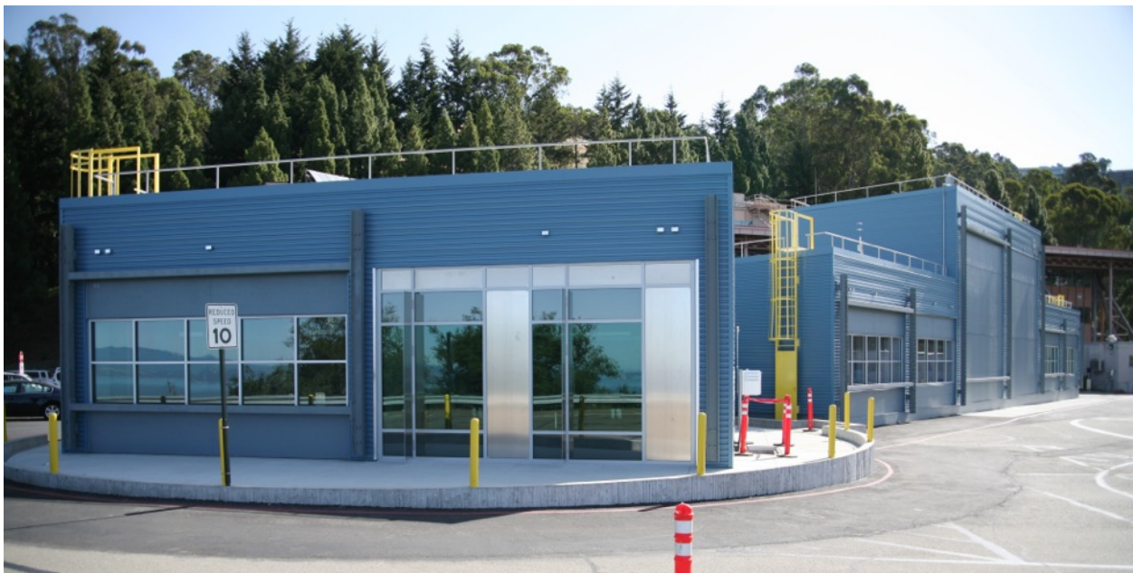
Figure 1.2 - Photo of DOE's FLEXLAB facility at LBNL. The B35 facade has been installed in the rotational test cell to the right in the photo.
