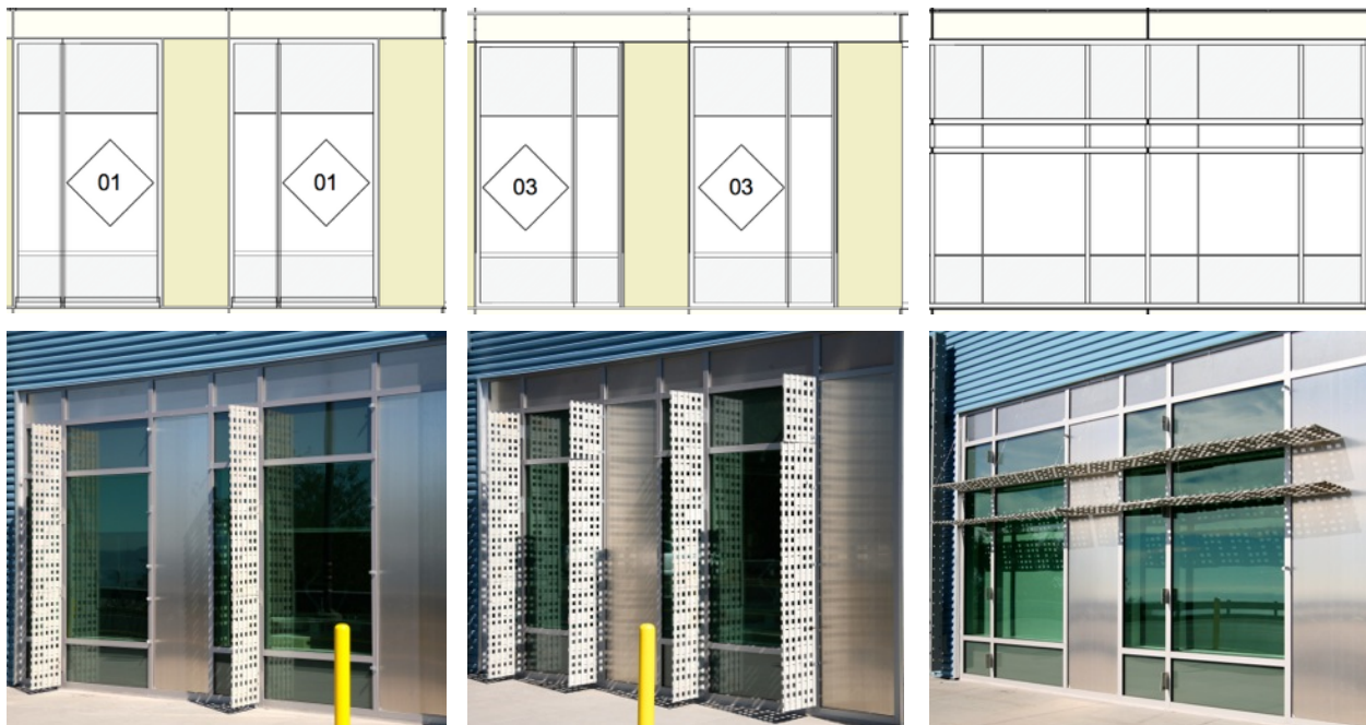
Figure 2.4 - Facade Elevations (top) and FLEXLAB configuration (bottom) for East facade (left) with one vertical fin per 10’ facade bay, West facade (center) with two vertical fins per 10’ facade bay and South facade (right) with two horizontal overhangs.
