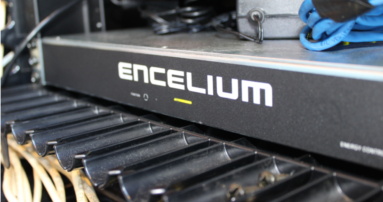
Figure 4.1 - Encelium's Rack mounted Energy Control Unit (ECU)
