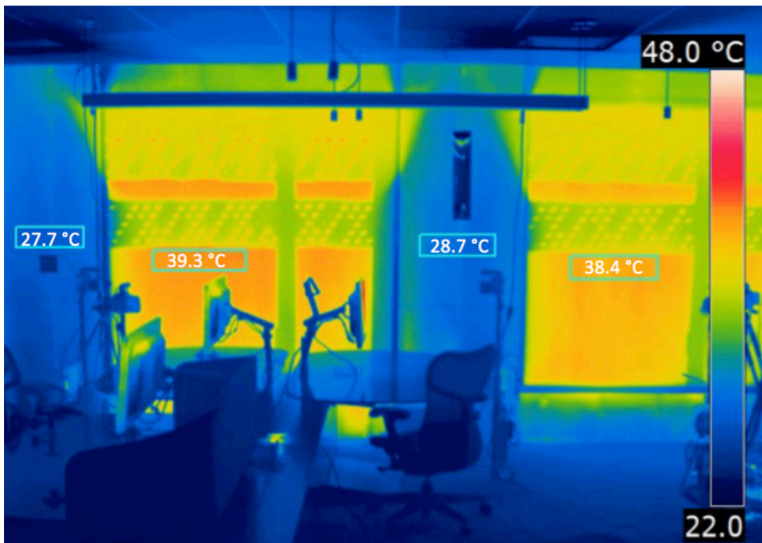
Figure 8.20 - Infrared Thermography image with shade deployed – October 6th 3:45pm PDT.
