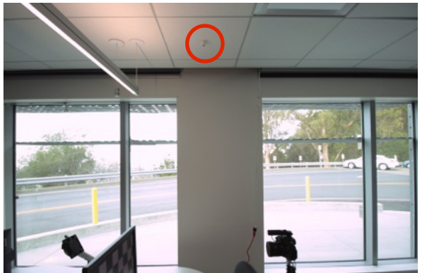
Figure 4.4 - Location of the Encelium photosensor (circled in red).
