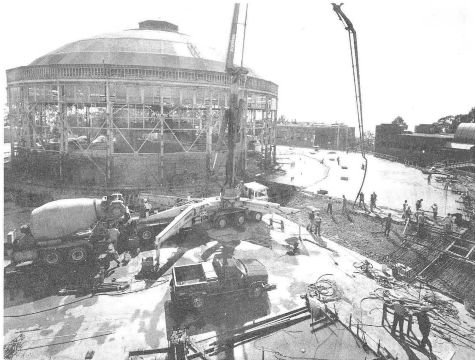
Five major pours totaling 4500 cubic yards of concrete were needed for the foundation and floor of the addition to Building 6. Consuming all of last summer, this work was completed last October 6, making way for erection of the new structural-steel framework.
