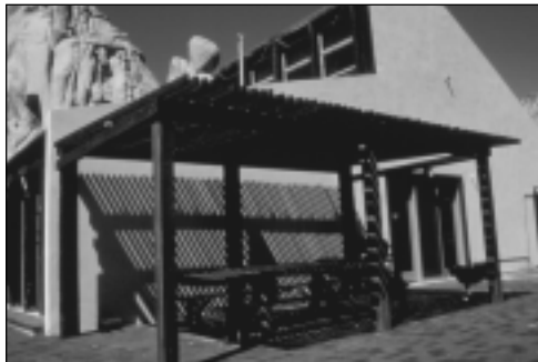
The Sibyl and Al A. Allanson Library and Center at Sweeney Granite Mountains Desert Research Center: (top) a distance shot showing the residence building and laboratory in their dramatic natural setting and (bottom) a closeup of the residence building. Photos by Jim André
