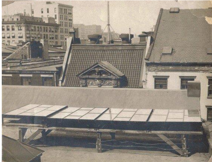
Figure 1.1.1 Image of the solar panel installed by Charles Fritts in 1883 on a New York City roof. 2
