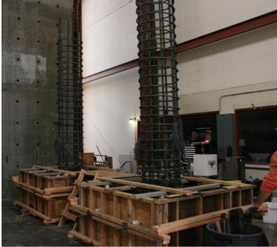
Figure 3.22 – Assembled forms for casting of footings
