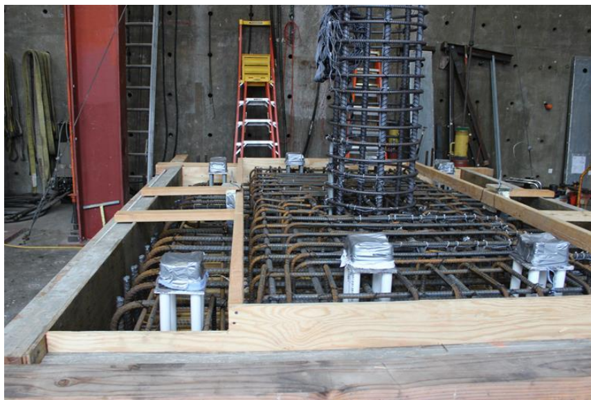
Figure 5.18 – Picture of slab and column reinforcement of Specimen #3 prior to cast
