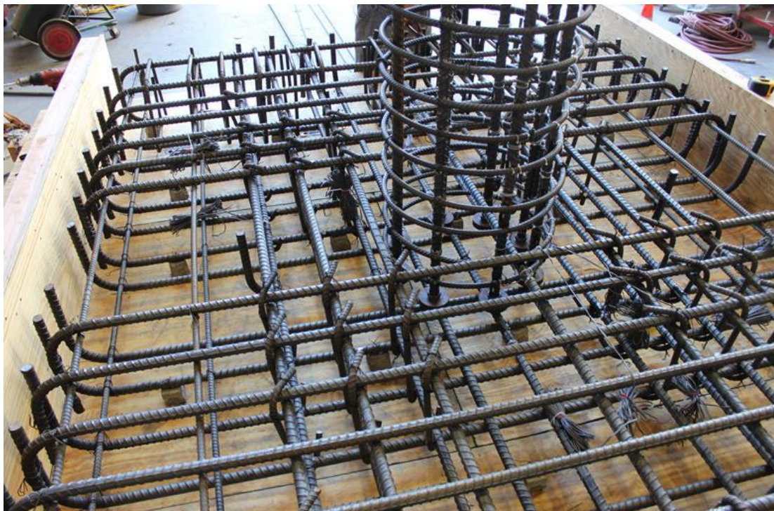
Figure 5.11 – Picture of the slab and column reinforcement of Specimen #1 during construction
