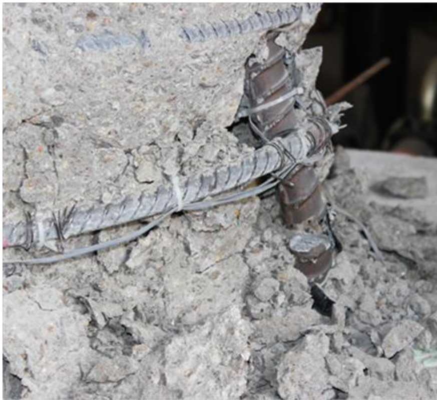
Figure 3.36 – Fractured bar 4 at north face of Specimen #1 during 2 nd cycle of -10% drift
