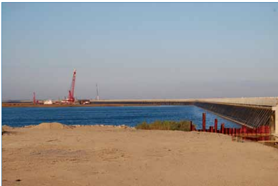
The Inner Harbor Navigation Canal surge barrier is the largest design-build civil works project ever awarded by the U.S. Army Corps of Engineers.
