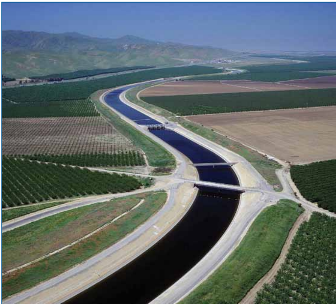
State Water Project Aqueduct, Central Valley, California
