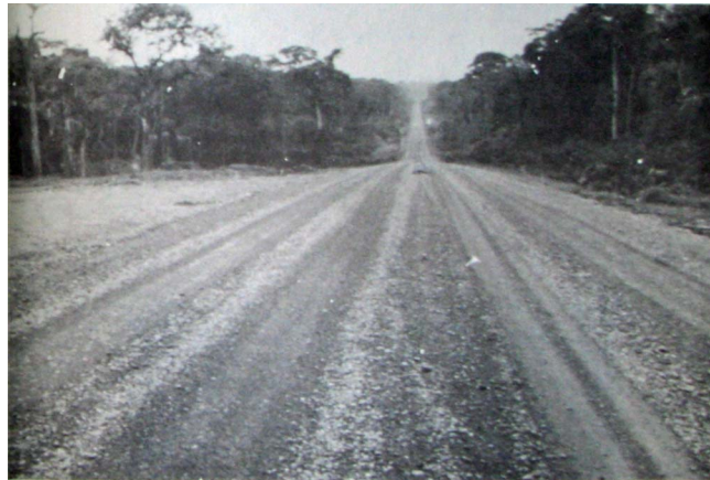
Figure 21. Official photograph from Ministry of Public Works, 1975 58
