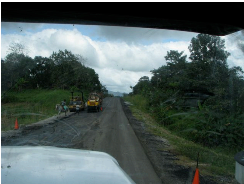
Figure 26. Compacting the road while two children and a horse walk through
