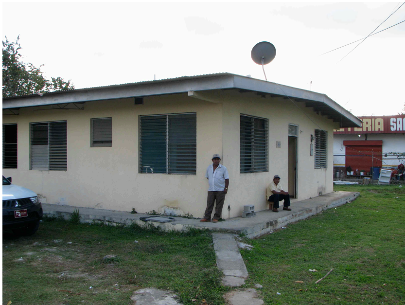
Figure 19. Former Emkay building in 2008, now part of the Ministry of Health's hospital facilities
