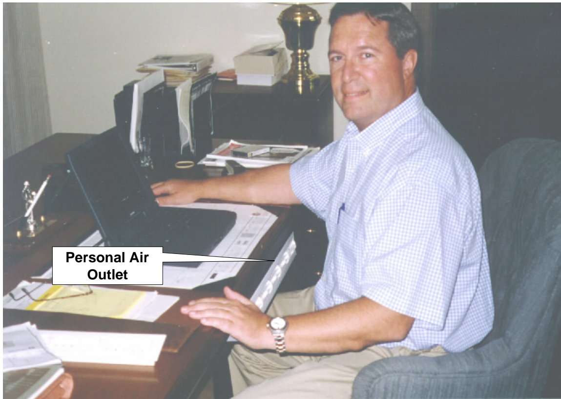
Figure 1. APACS Personal Air Outlet mounted horizontally under desk
