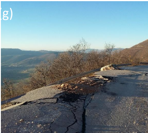
Figure 4.79. Fracture along the road, large vertical offset due to fracture and ultimate movement, damaged edge barriers and debris and boulders on the road surface.
