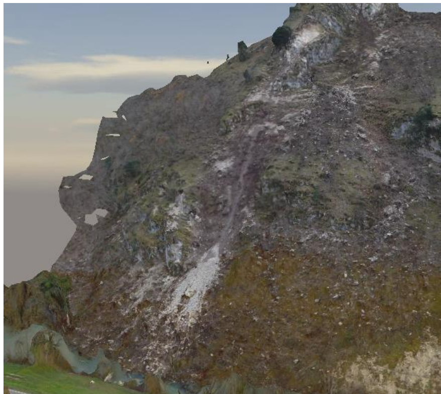
Figure 4.62. Lateral view from the drone of the rock column at km 3 of SP134 (right valley flank) (a). The left part of the column cap collapsed producing two small avalanches towards the column front and along the column free side. Scars left from two wedges on the adjacent cliff (b). Leftward tilting of the column cap is also visible in figure 4.61.
