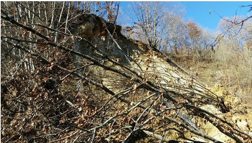
Figure 4.102. Landslide debris and head scarp. Also pictured is rockfall netting.
