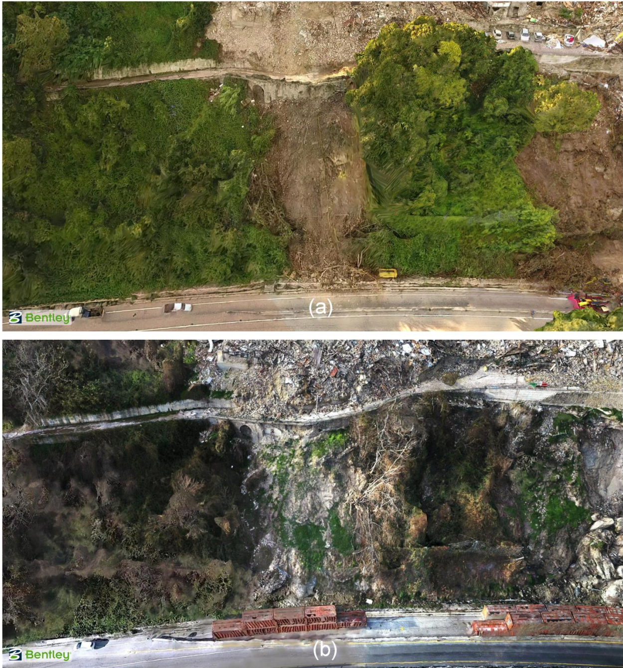
Figure 4.23. 3D model comparison of the smaller landslide below Pescara del Tronto between September 2016 (a) and December 2016 (b).
