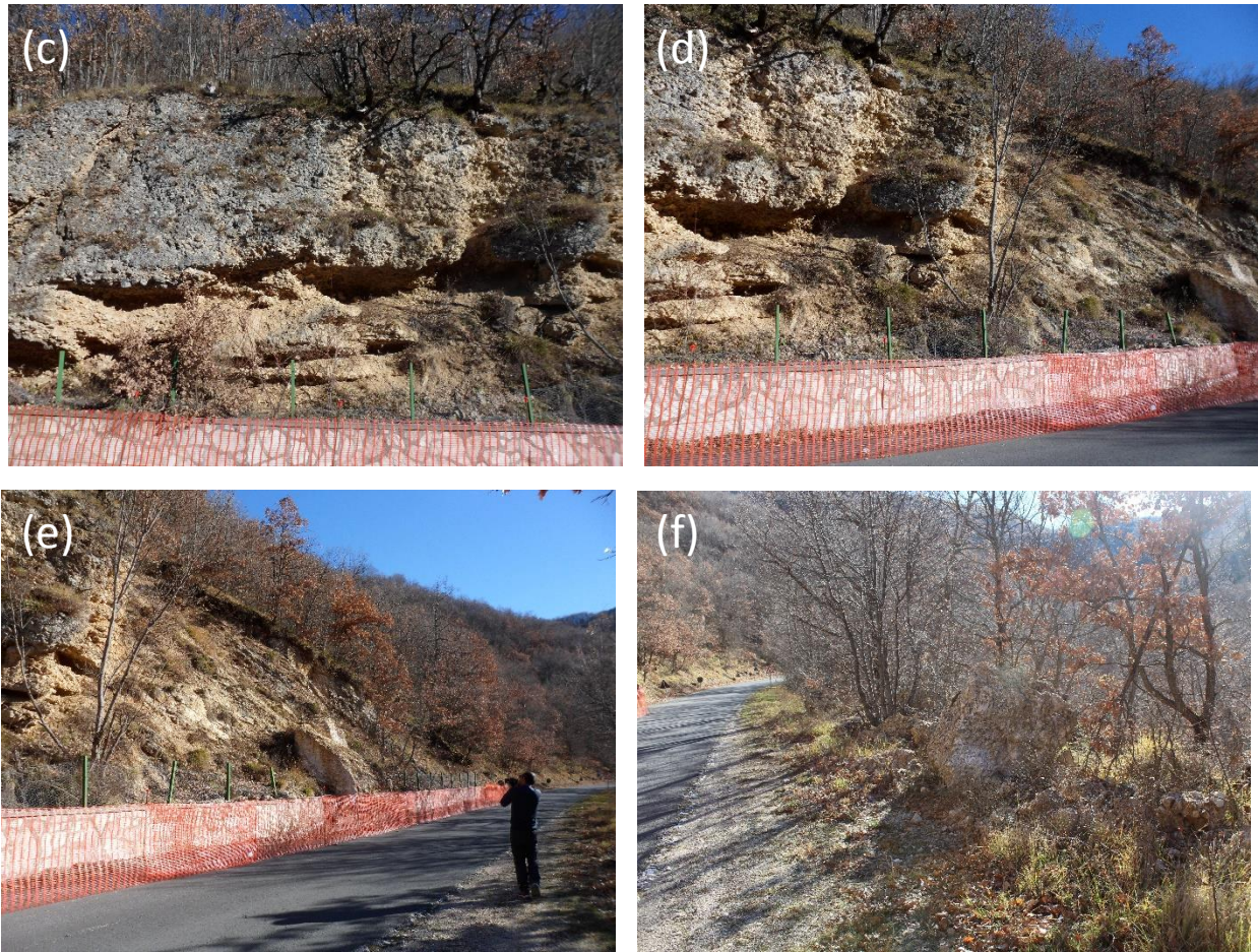
Figure 4.89. Failure in calcareous breccia between Cittareale and Norcia along the SP746: from (a) to (e) view of the all facade; (f) rockfall on the road.
