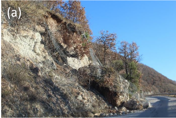
Figure 4.77. Debris and boulders captured by the rockfall protection nets.
