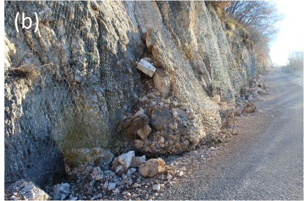
Figure 4.77. Debris and boulders captured by the rockfall protection nets.
