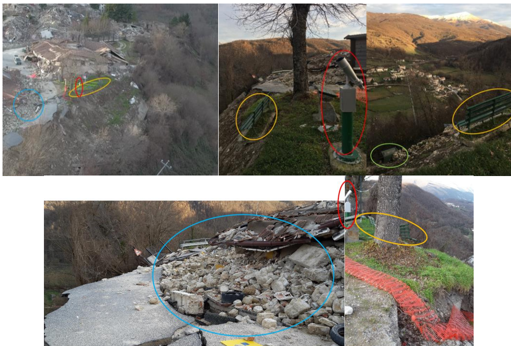
Figure 6.27. Representative pictures of landslide in the eastern part of village (December 2016).
