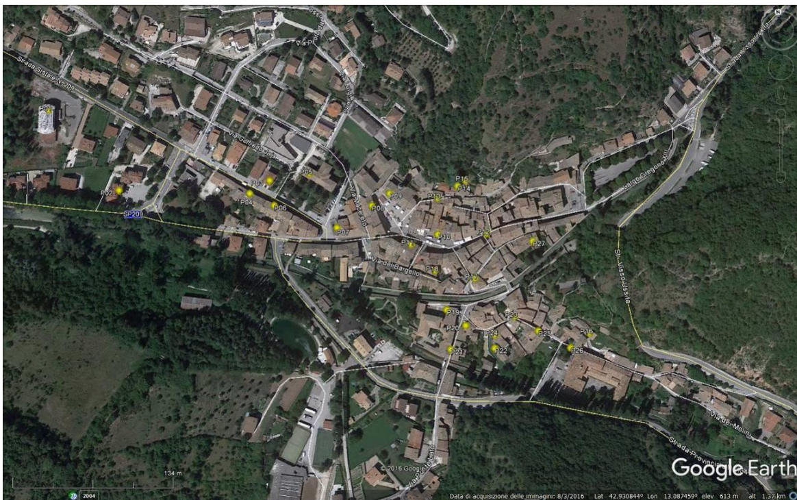
Figure 6.65. Locations of representative structures inspected in the Visso village (see Table 6.8 for details).
