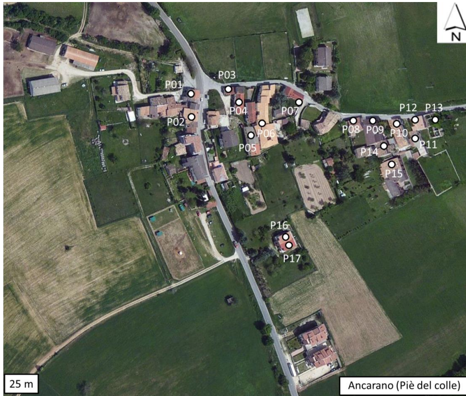
Figure 6.104. Locations of the representative structures inspected in Ancarano piè del colle (see Table 6.16 for details).
