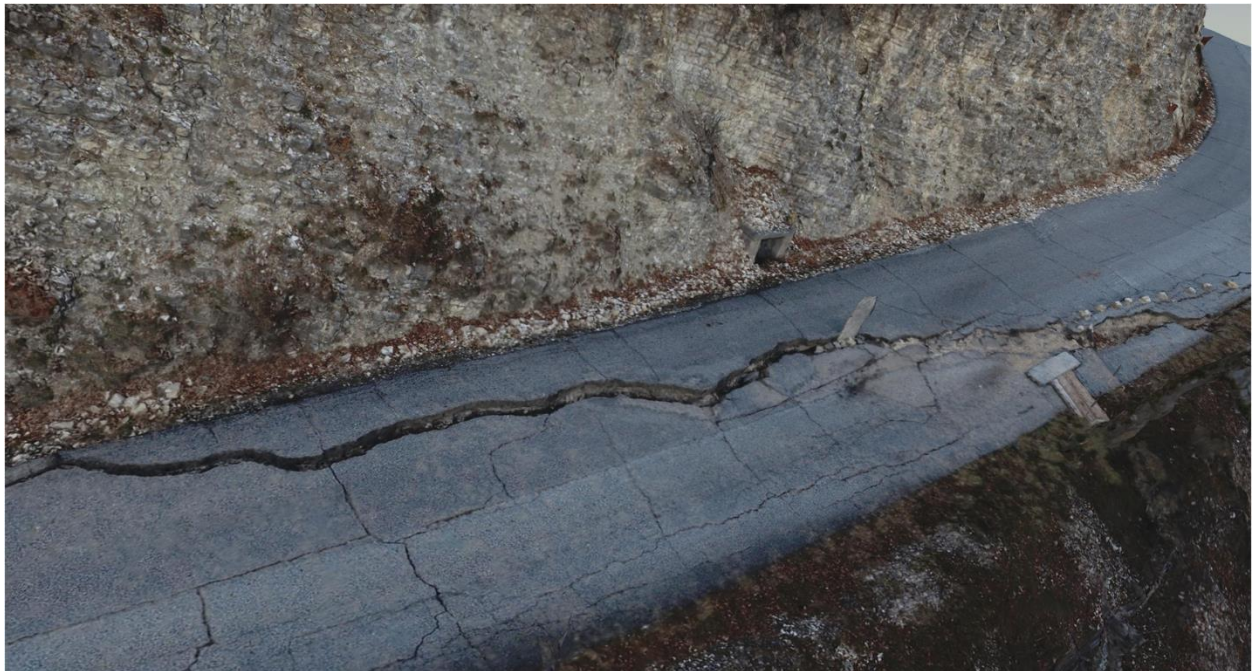
Figure 4.38. 3D model of the eastern half of the Valle di Panico landslide headscarp.
