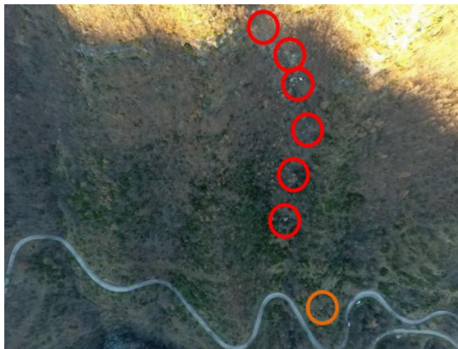
Figure 4.47. UAV aerial image of rockfall path from source at top of slope to the road at bottom of slope. Red circles show boulder fragments larger than 1.5m. Last boulder fragment from rockfall near road at base of slope is circled in orange.
