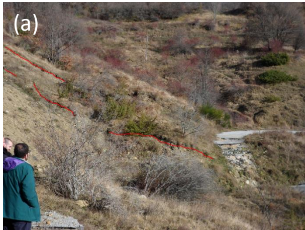
Figure 4.94. Fractures on the cut slope.
