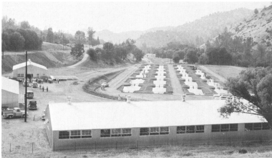
FIGURE 50. Moccasin Creek Hatchery on the day of dedication, June 29, 1954. The initial installation included 24 standard raceway ponds. Twelve additional ponds were added in 1955.
