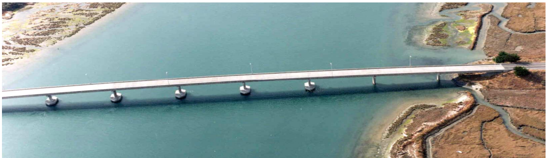
Figure 2.1: Humboldt Bay Middle Channel (HBMC) Bridge (Courtesy of Caltrans)
