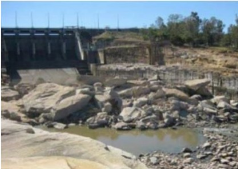
Fig. 1. Removal of large rock blocks from unlined spillway at Wivenhoe Dam in Australia (Stratford et al., 2013). For scale, spillway width is approximately 90 m.
