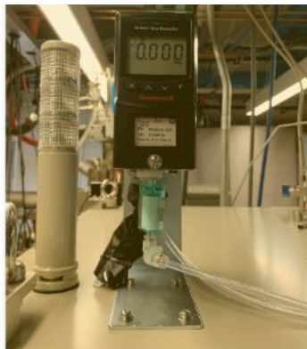
Figure C.1. The ozone sensor for monitoring leaking inside POG
