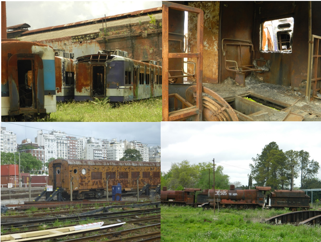
Figure 14: Rusted rolling stock in Liniers (top two), Retiro (bottom left), and Empalme Lobos (bottom right). Photos by author.
