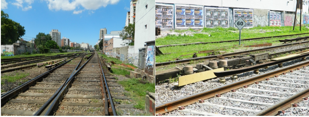
Figure 15: Wooden (left) and concrete (right) crosssties near Caballito station, on the Once-Moreno branch of the Sarmiento line. The stretch of tracks on the right has been “renovated”, while the stretch on the left has not, presumably because the latter is a zona de cambios, a track-switching area. Track-switching areas see a higher number of derailments and thus need to be repaired/intervened more often; wooden crosssties, being lighter, are easier to maneuver by a track maintenance crew, without requiring heavy-lifting machinery. Photos by author.
