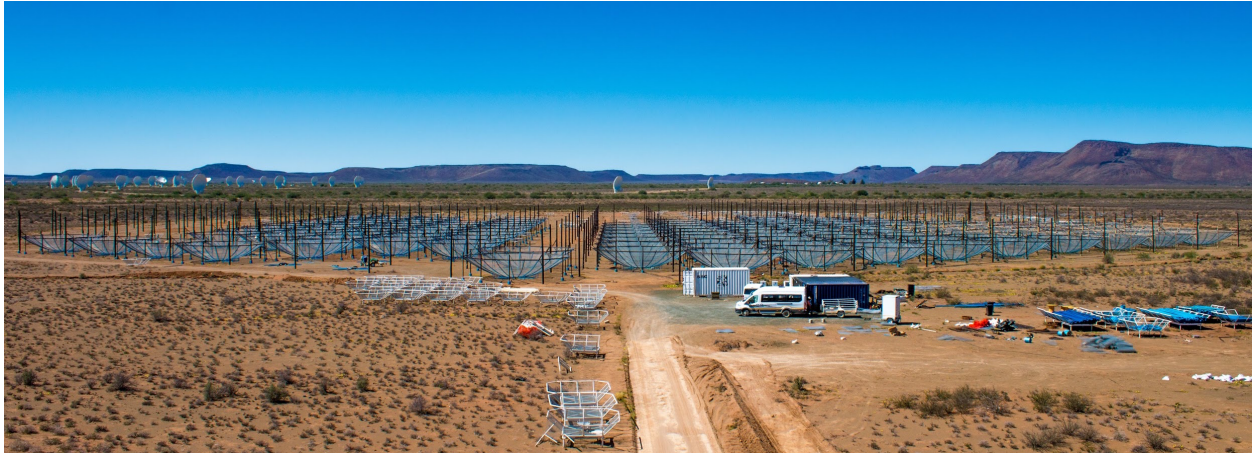
Figure 1.4: The Hydrogen Epoch of Reionization Array (HERA) in the Summer of 2018. Over 100 dishes have been built with old original feeds.
