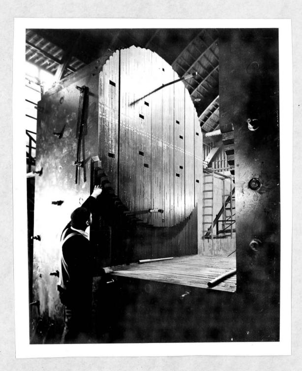
Fig. 7. Another View of the Complete Magnet of the 90-inch Cyclotron.
