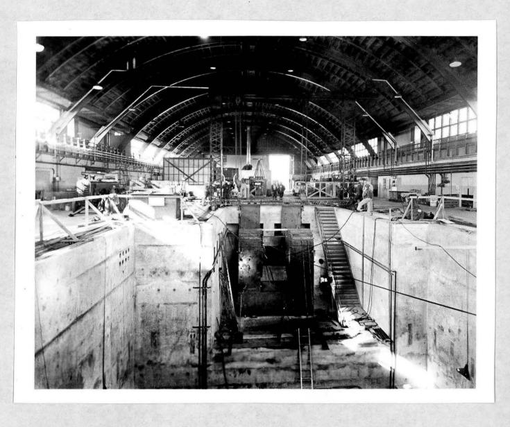
Fig. 4. The Magnet Yoke of the 90-inch Cyclotron.
