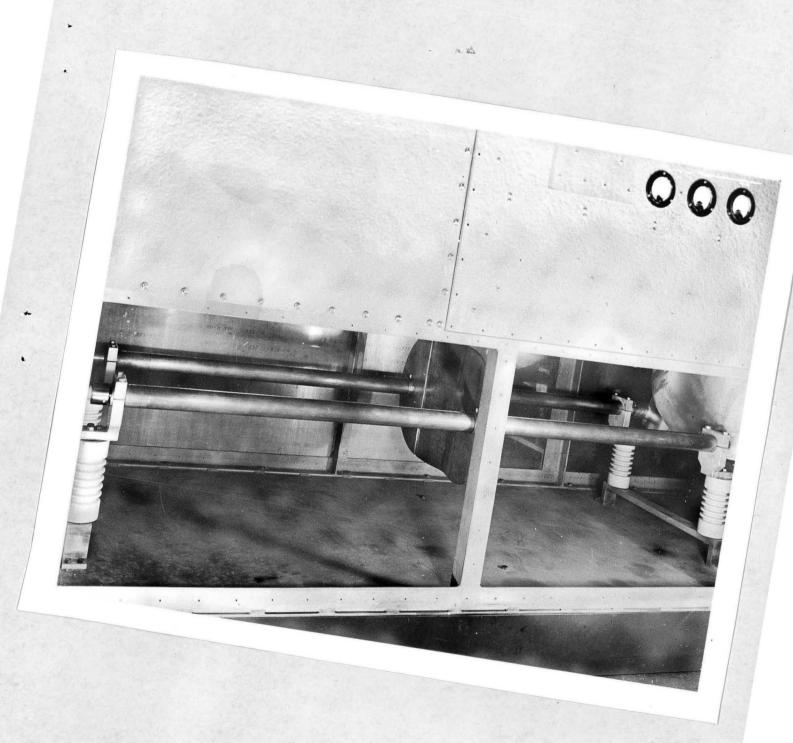
Fig. 10. The Grid Resonator of the Final Amplifier. The position of the shorting plane is adjusted by means of lead screws within the grid lines.
