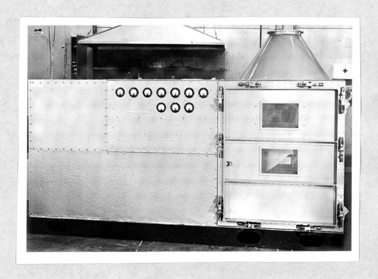
Fig. 8. The Driver and Final Amplifier of the 90-inch Cyclotron
