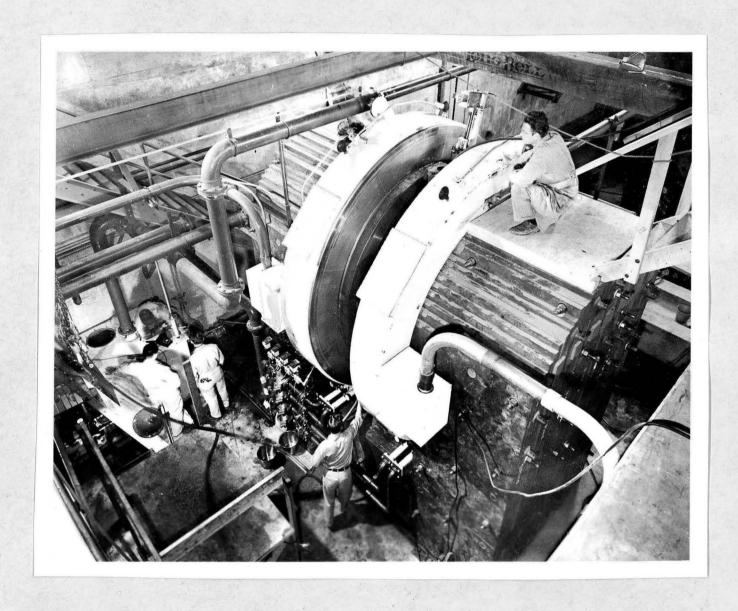
Fig. 6. The Complete Magnet of the 90-inch Cyclotron.
