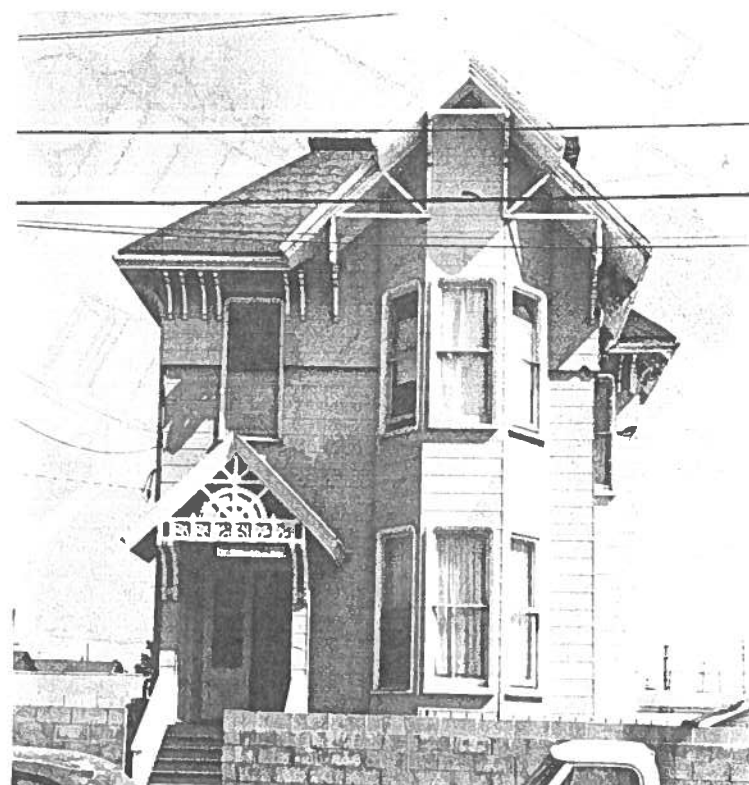
Adjacent to site on 7th Ave.
