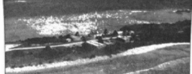
Aerial view shows strip of land on Hagres where test warheads come crashing down after 4,950-mile trip from Vandenberg Air Force Base.
