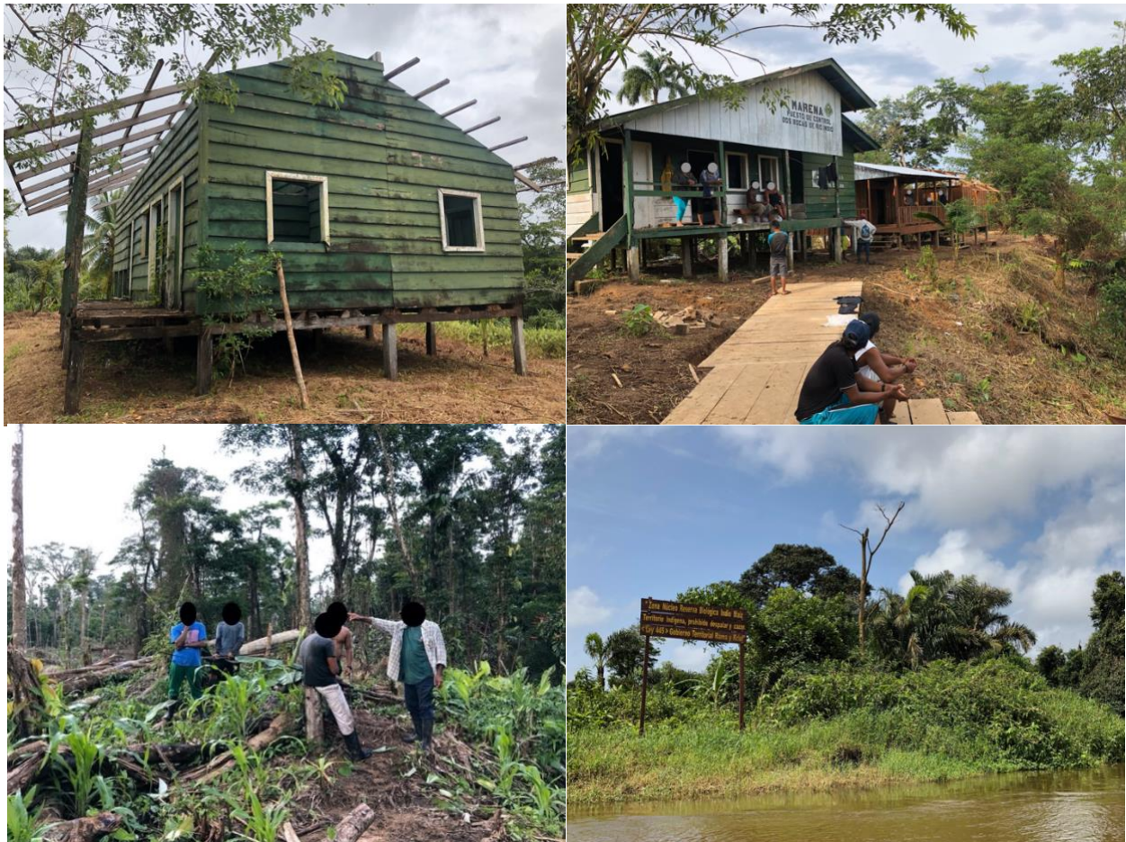
Figure 3 (top left): The abandoned, deteriorating military post at Dos Bocas. Figure 4 (top right): The old MARENA control post (left) alongside construction of new communal forest ranger station (right) at Dos Bocas. Figure 5 (bottom left): A Rama communal government member (far right) and two community members armed with bows and arrows (far left, center-left) inform two new settlers (center, center-right) that they have deforested communal lands in a protected area and must leave. Figure 6 (bottom right): A sign installed by communal forest rangers reading, “Core area, Indio-Maíz Biological Reserve. Indigenous territory, deforestation and hunting prohibited. Law 445. Rama-Kriol Territory Government.” Photos by author, 2019.
