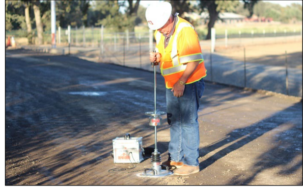
Figure 4.9: Testing with light weight deflectometer.
