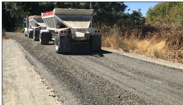
Figure 5.3: Shaped road prior to recycling.
