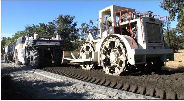
Figure 5.8: Primary compaction with a segmented padfoot roller.
