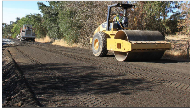
Figure 5.10: Final compaction with a smooth drum roller.
