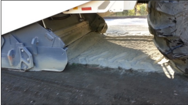
Figure 2.10: Cement redistribution in front of mixing chamber.
