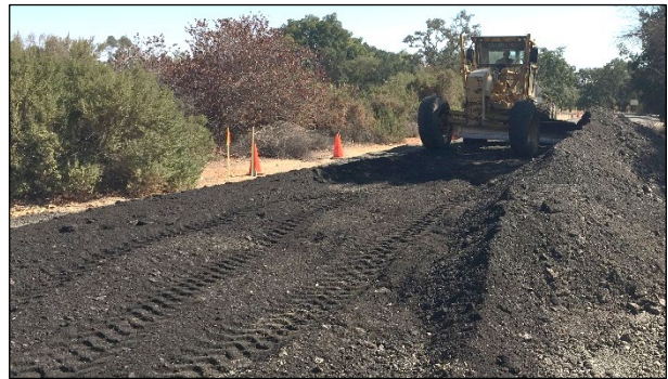
Figure 5.2: Spreading imported RAP.
