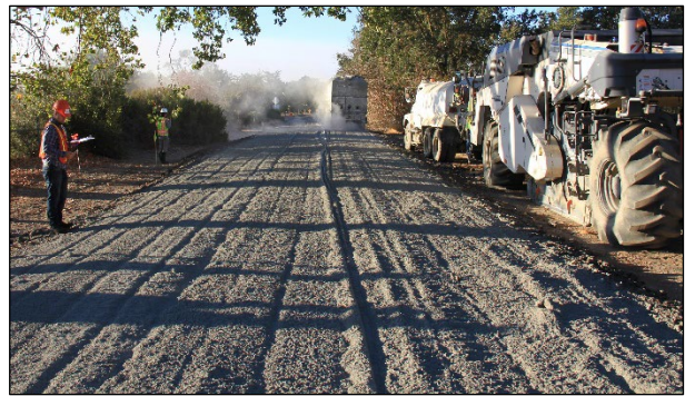
Figure 5.5: Checking cement spread overlaps.
