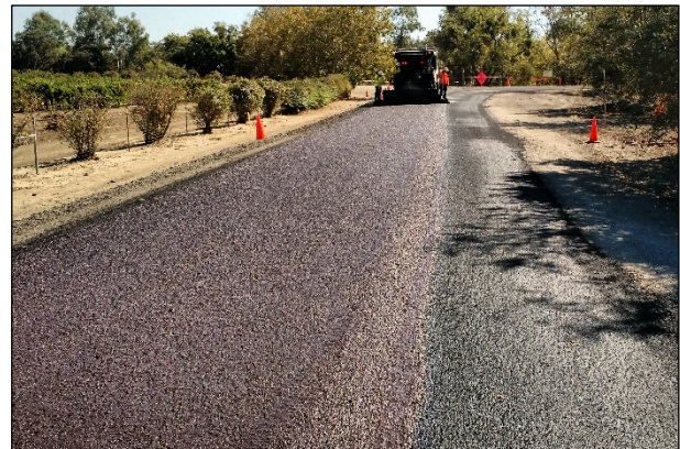
Figure 5.38: Second microsurfacing pass.
