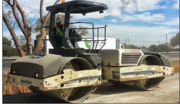
Figure 4.5: 10-ton DSR roller used for microcracking on FDR-C Test Road.
