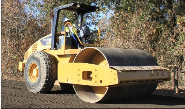
Figure 4.4: 12-ton SSR used for microcracking on FDR-C Test Road.
