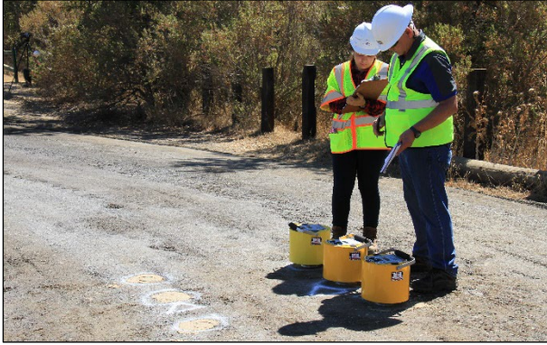
Figure 4.8: Testing with soil stiffness gauges.
