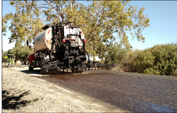
Figure 5.36: Prime coat application.
