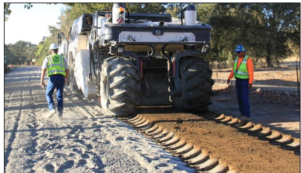
Figure 5.7: Recycled material behind the reclaimer.
