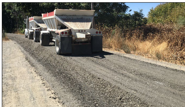
Figure 5.3: Shaped road prior to recycling.
