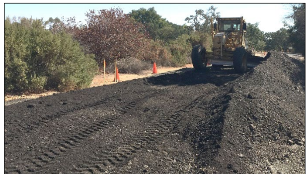
Figure 5.2: Spreading imported RAP.
