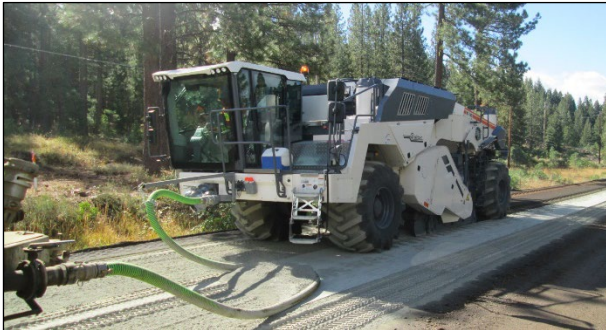
Figure 2.7: Hose dragging cement.
