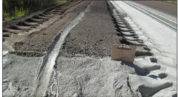
Figure 2.11: Accumulation of cement at end of recycling section.
