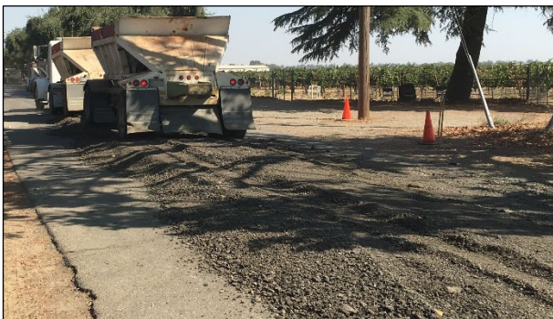
Figure 5.1: Dumping imported RAP.
