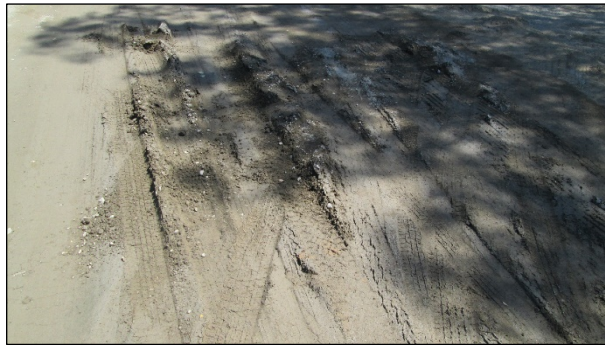
Figure 2.9: Wet spot from spill still visible after final compaction.
