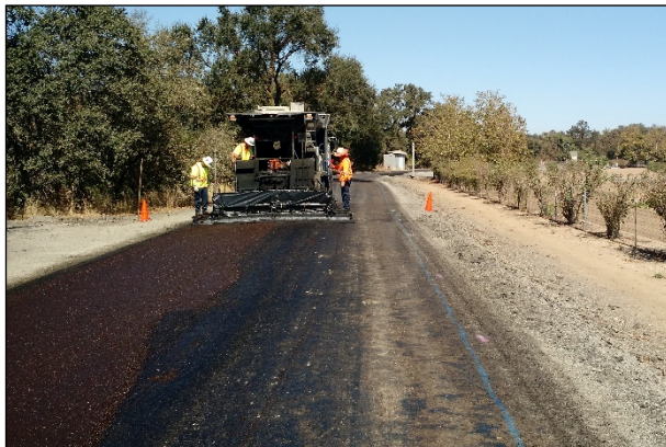
Figure 5.37: First microsurfacing pass.
