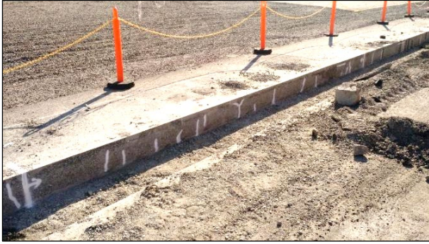
Figure 2.26: Dry FDR-C test section.
