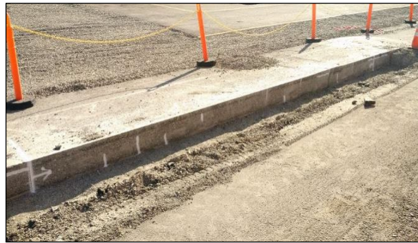
Figure 2.28: Wet FDR-C test section.
