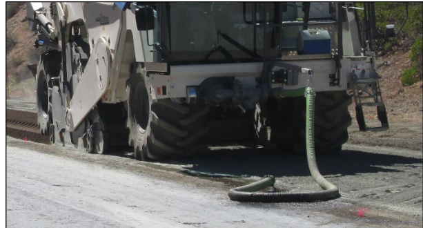
Figure 2.8: Water spill during tanker change.
