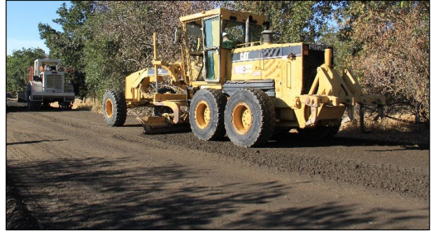
Figure 5.9: Leveling with a grader.
