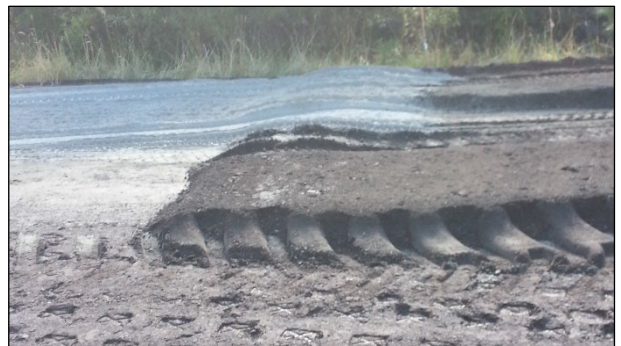
Figure 2.13: Cement spreading overlaps.
