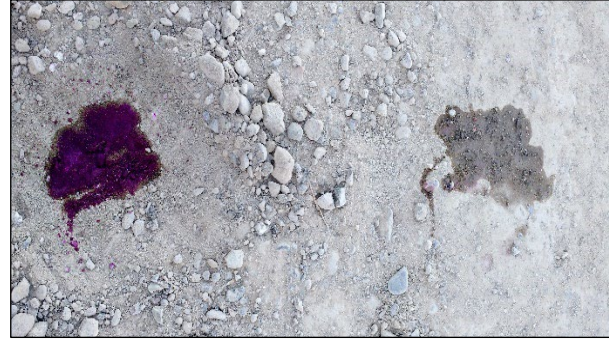
Figure 3.5: Surface carbonation on an FDR-C layer.
