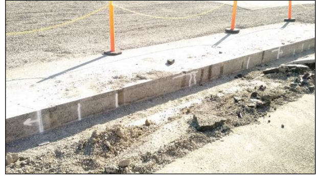
Figure 2.27: Area between dry and wet test sections.
