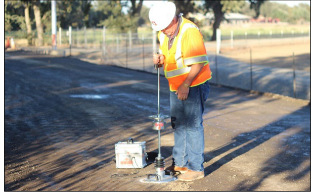
Figure 4.9: Testing with light weight deflectometer.
