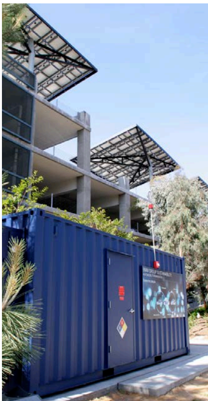
Photo of University of California San Diego (UCSD) second-life EV battery project facility
