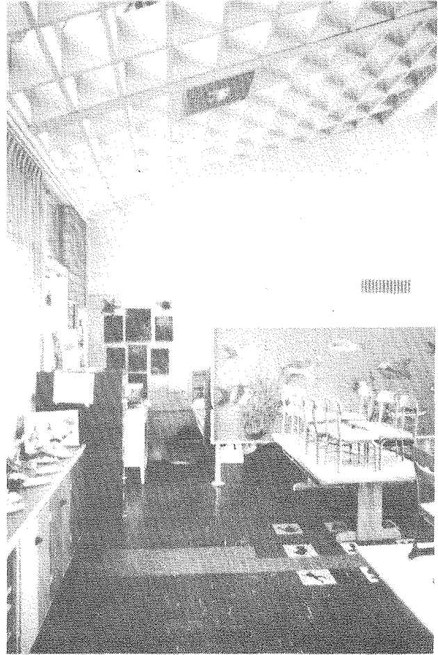
Daylighting design for schools produced many innovations during the 1950s. In the Mira Vista Elementary School, daylight is diffused through a grid in the classroom ceiling. The grid, in addition to diffusing the light, reduces light contrasts that might cause visual discomfort.
