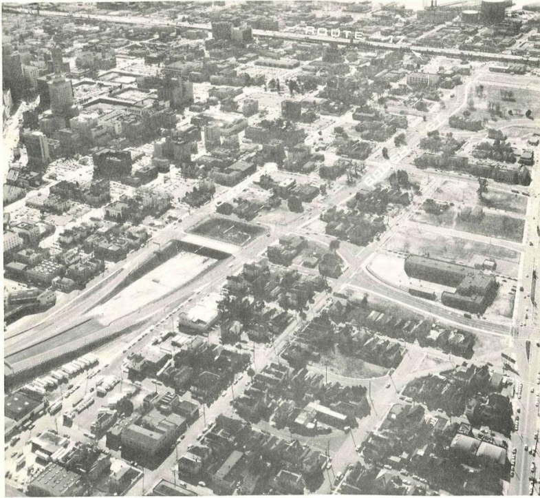
PROJECT AREA LOOKING SOUTH
