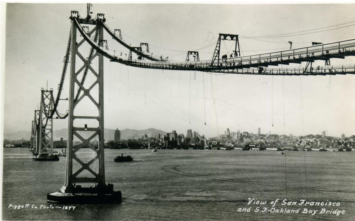
Figure 25: San Francisco-Oakland Bay Bridge from Yerba Buena Island during construction
