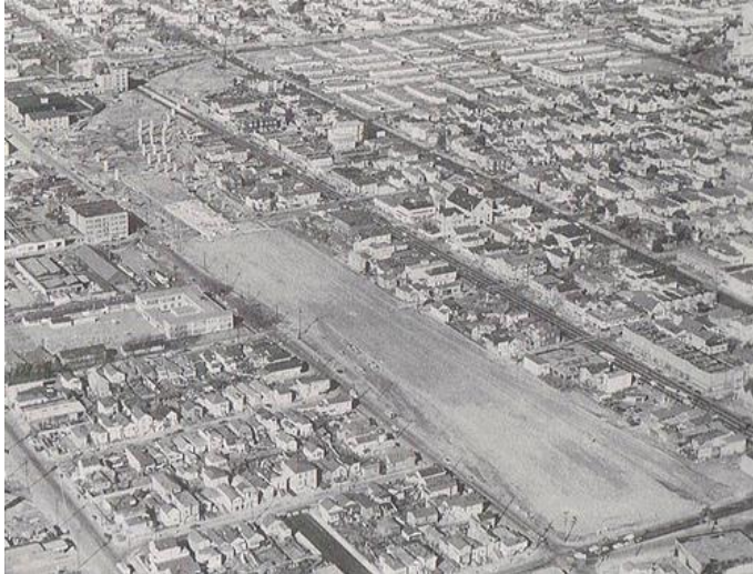
Figure 1: Demolition for the cypress freeway in West Oakland
