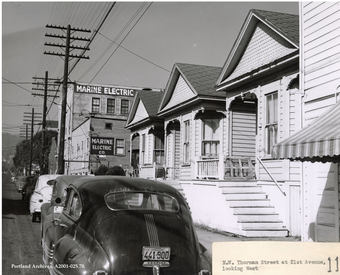
FIGURE 4-9: The Vaughn Area at midcentury was a mixture of uses, with homes dating to the 19 th century interspersed with industrial uses that dated to the 20 th century. The result was that when new industry was built in this area, it was butted up against home uses, but also was restricted in its overall size based upon available lots sized originally for houses, not factories. The Planning Commission, in selecting the Vaughn area for redevelopment, hoped to clear these homes from the urban landscape entirely, in order to assemble larger lots for the location of larger, more modern industrial uses. Here, then, the
