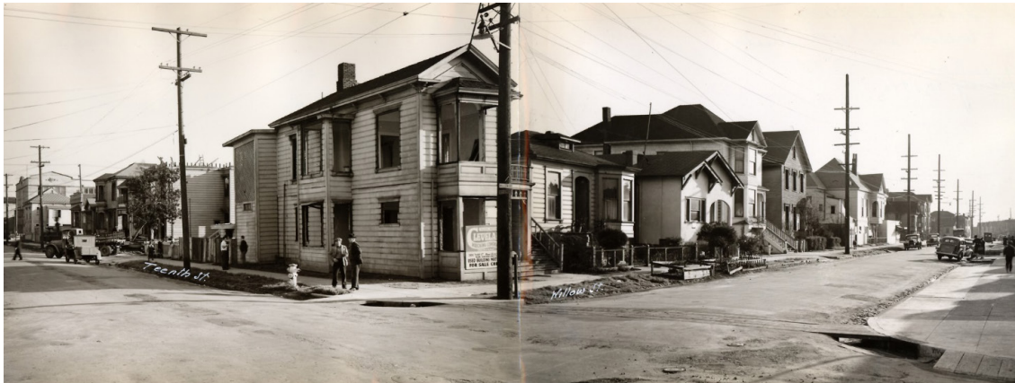
FIGURE 3-3: 10 th and Willow Streets in West Oakland, looking southeast at future location of the OHA's Campbell Village project. Even with early demolition underway, the street looks handsome, clean, and reasonably maintained. There is not even evidence of land use mixing such as industrial encroachment or jury-rigged retail uses. Moses L. Cohen for the Oakland Housing Authority, January 10, 1940. Oakland Housing Authority collection, Oakland Public Library, copl_079.
