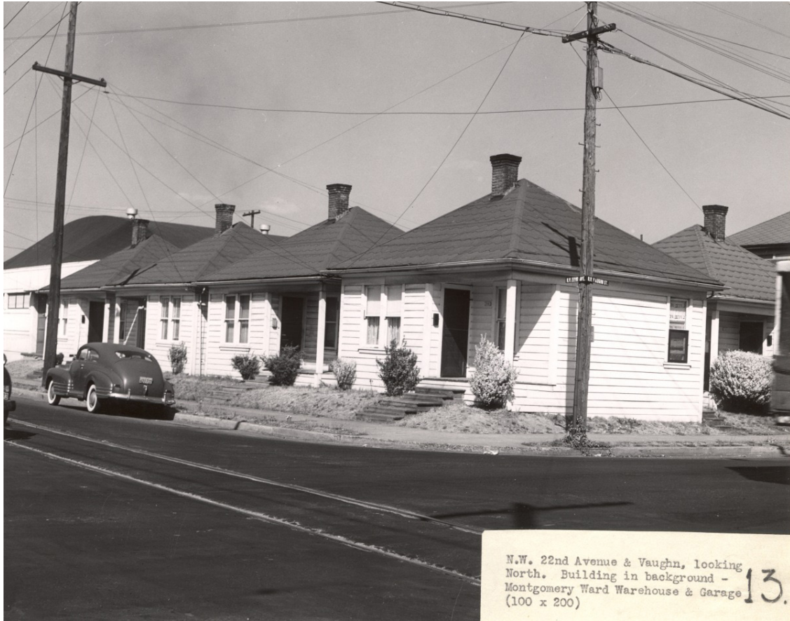
FIGURE 4-10: This is an example of the kind of land use that HAP's redevelopment board considered to be blight. The arch-truss building in the background was a supplementary warehouse for Montgomery Wards, whose main facility was located at 27th and Wilson, five blocks west and marking the westernmost border of the Vaughn Street Redevelopment Area. Expansions of industrial uses into the project zone had
