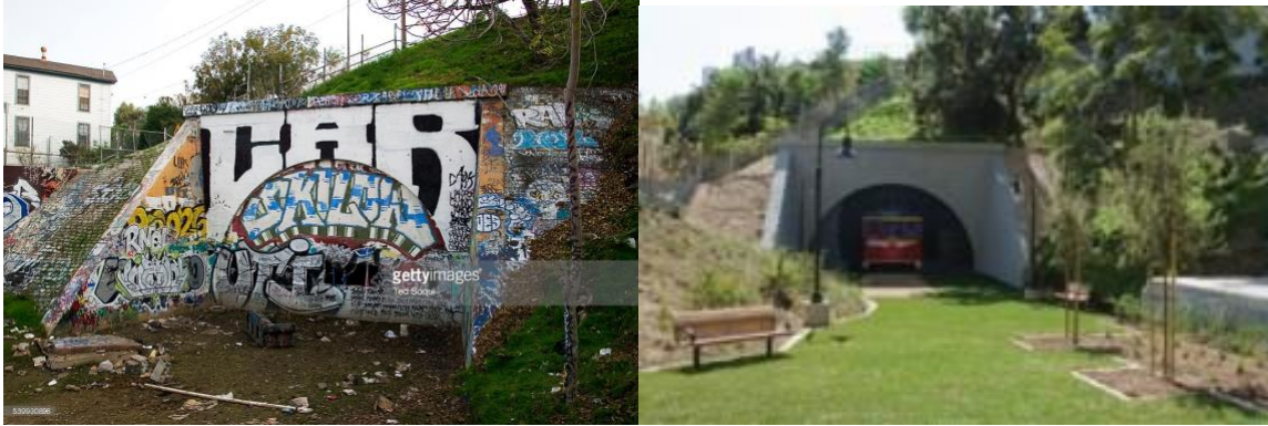
(Image 5. Belmont Tunnel before and after. http://www.gettyimages.com/detail/news-photo/the-entrance-to-the-belmont-tunnel-a-haven-for-graffiti-news-photo/539930896#the-entrance-to-the-belmont-tunnel-a-haven-for-graffiti-artists-for-picture-id539930896 )
