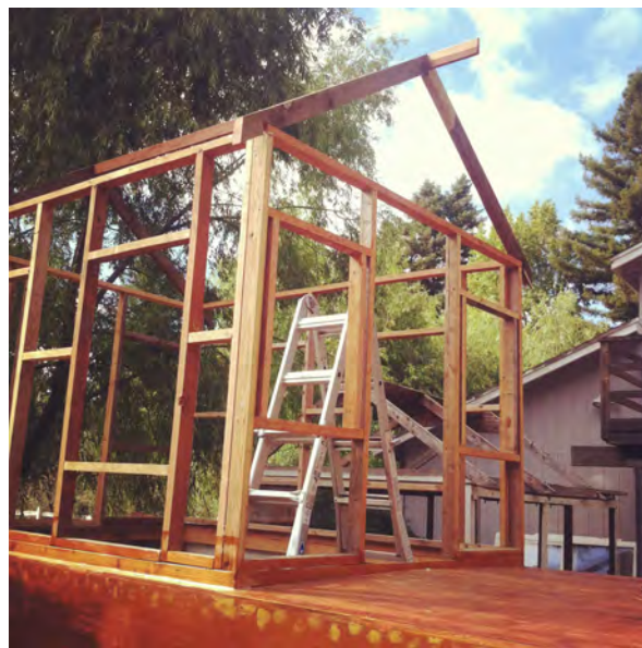
Figure 7. Shantyboat cabin framing.
