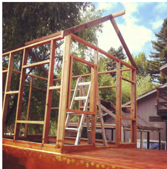
Figure 7. Shantyboat cabin framing.
