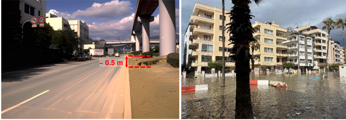
(a) (b) Figure 5.1. (a) Post-liquefaction free-field settlement at Port Island after the 1995 Kobe earthquake (Akai et al. 1995), and (b) Flooding of the inland street and buildings in Iskenderun after the 2023 Türkiye earthquake (Photograph from the GEER 2023 reconnaissance).
