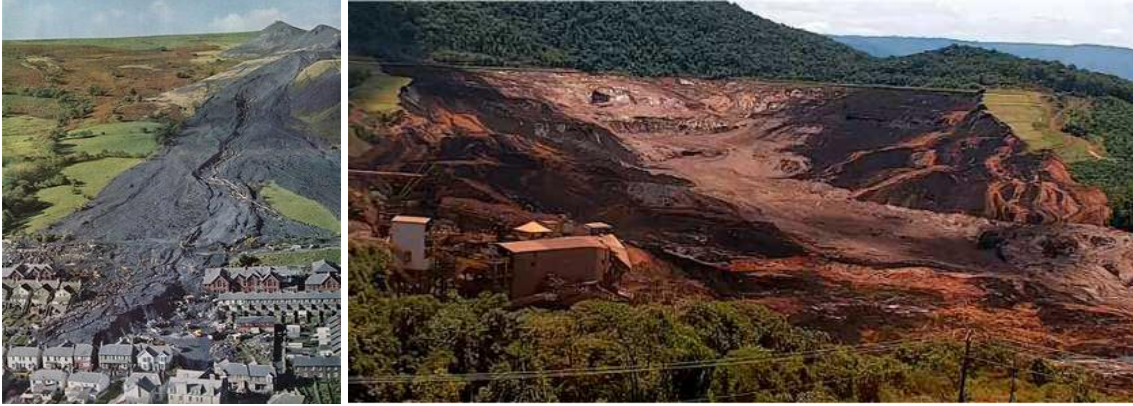
Figure 6.1. (a) 1966 Aberfan, UK slope failure that killed 144 people, which was attributed to constant shear drained stress path loading (Stava Foundation 2021), and (b) Fundao tailings dam failure (Morgenstern 2016).
