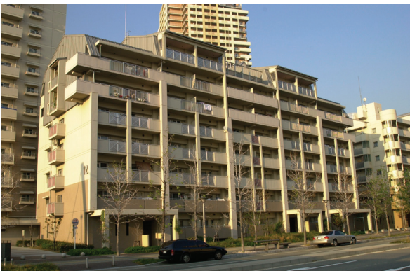
Figure 2 : Public housing in Kobe
