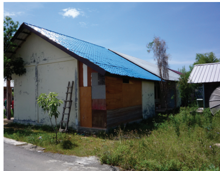
Figure 1: This ADB house is shown right in its unmodified form. The plan on the left shows the modified house with the most simple of additions. Timber framed and plywood clad walls have been added to the porch at the rear of the house. The existing concrete slab and roof made this an inexpensive modification that now provides residents some privacy when entering the bathroom as well as security for their cooking equipment Source for all figures: David O'Brien
