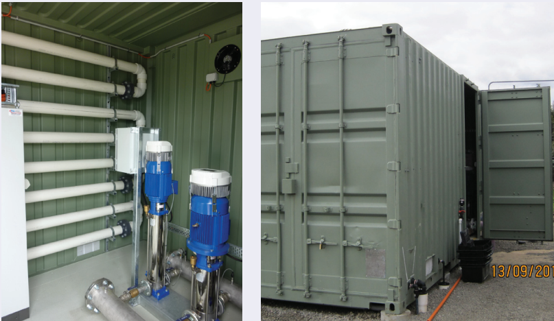
Figure 2: A mobile water treatment system is one possible temporary infrastructure use for shipping containers
