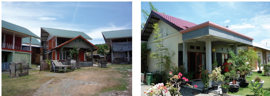
Figure 6: The heads of both of these households have prominent positions in government (policeman and administrator) as well as in their community. The façades of their houses reflect this – on the left we see a substantial new front portico added to a Bank Mandiri house and on the right we see an ADB house with a new portico that includes highly decorated front doors, a façade lined with tiles and decorative plants in the garden
